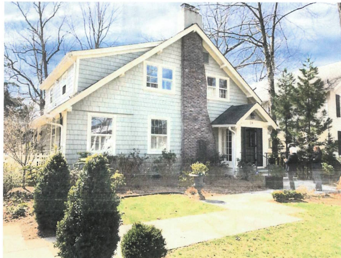
NORTH FACADE, FROM PUBLIC ROW
