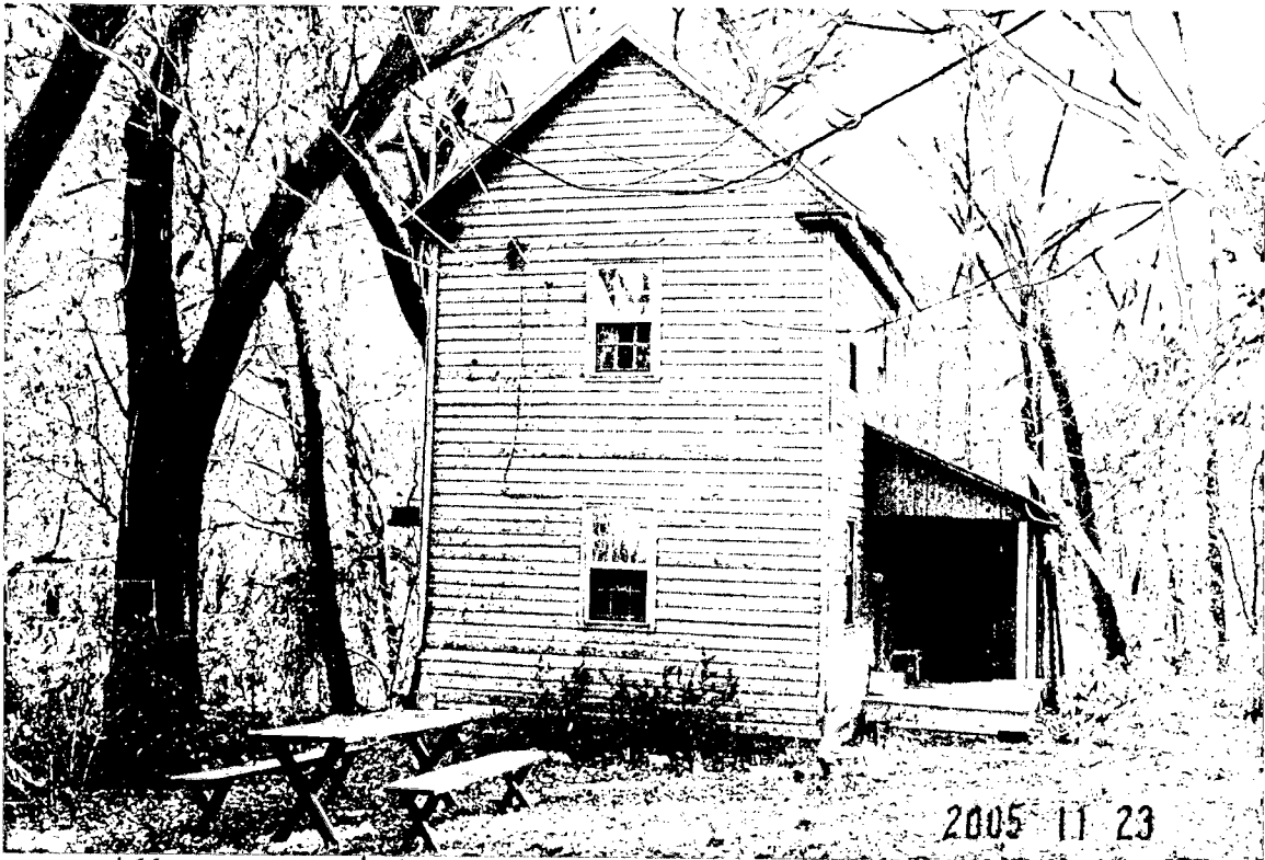
WEST SIDE VIEW OF TENANT HOUSE
