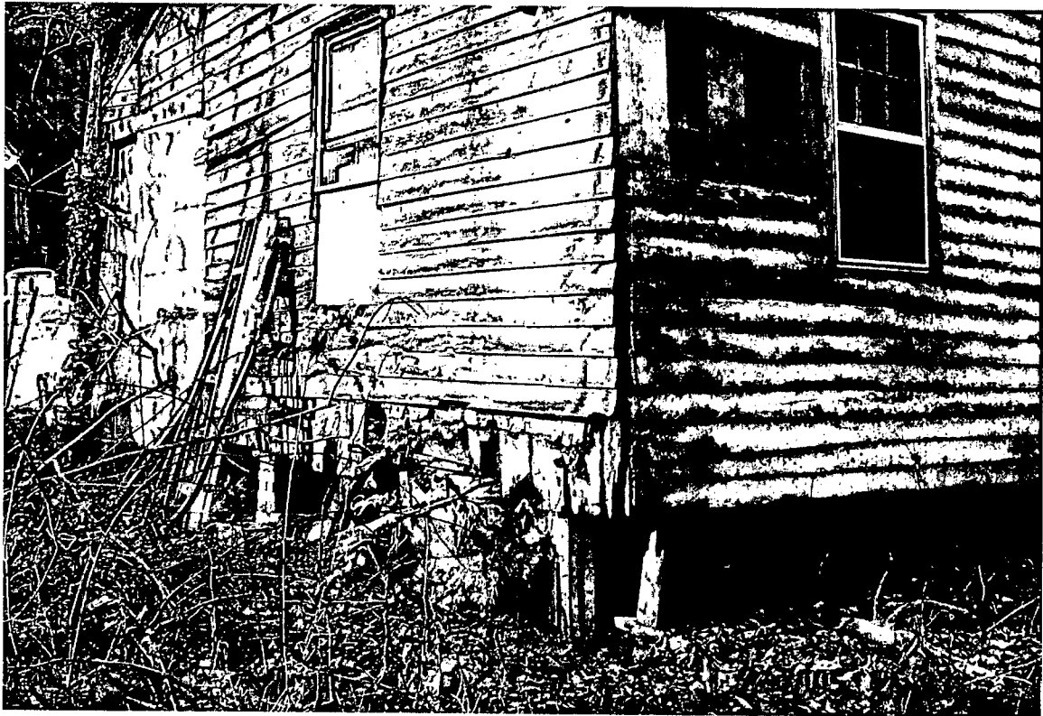
NORTH EAST CORNER OF TENANT HOUSE
