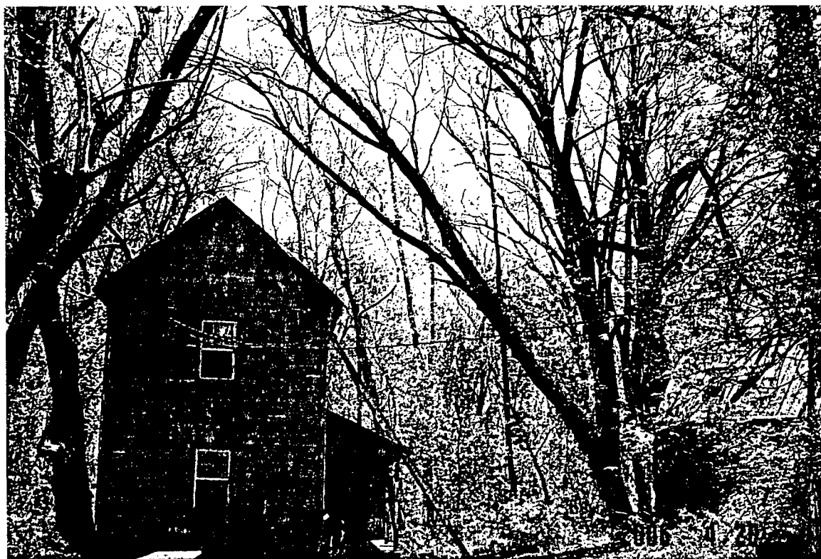
WEST SIDE VIEW OF TENANT HOUSE
