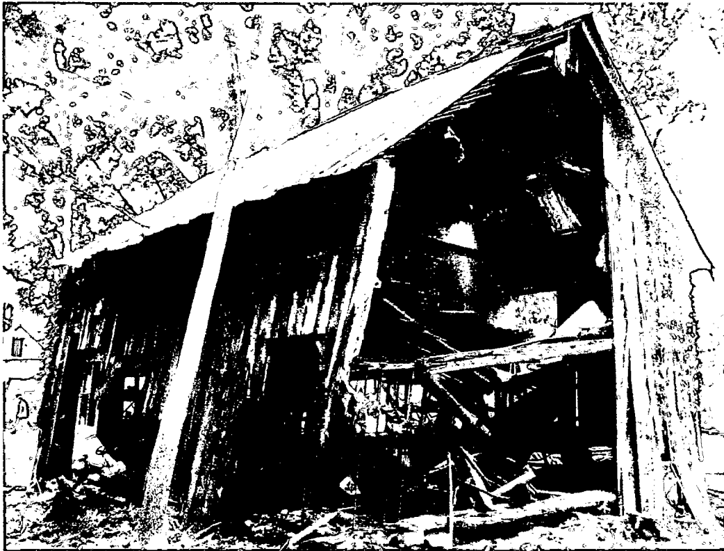
South East Corner
