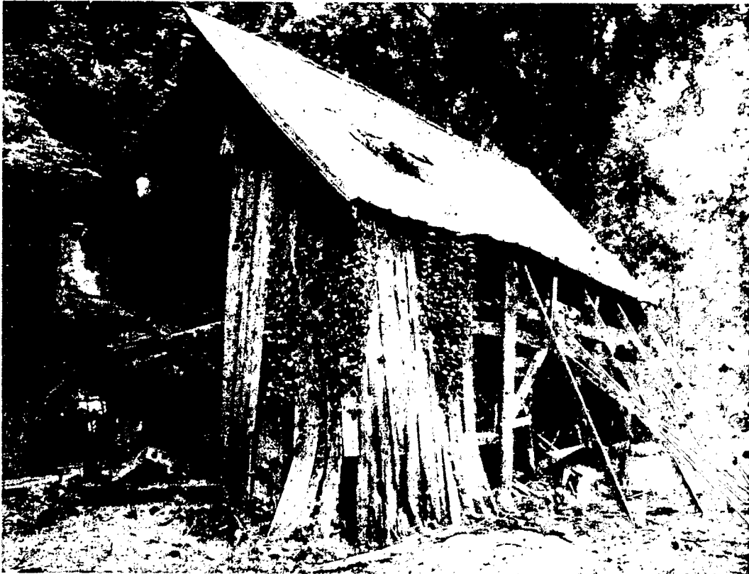
North East Corner, (starting stabilization)
