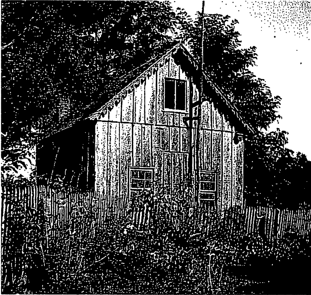
West Elevation Blacksmith Shop Photo from Jim Stabler, date unknow
