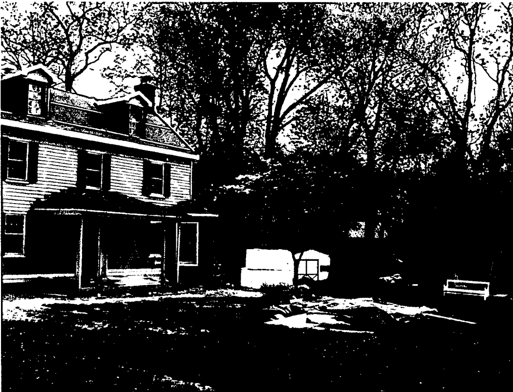
View looking East, blacksmith shop on far right, 125' East of main house, behind bench and tree
