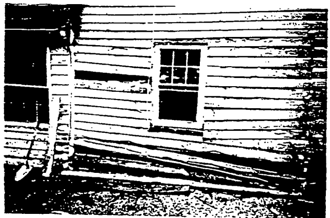
f.jpg Detail of Structural Problems. Foundation is crumbling.
