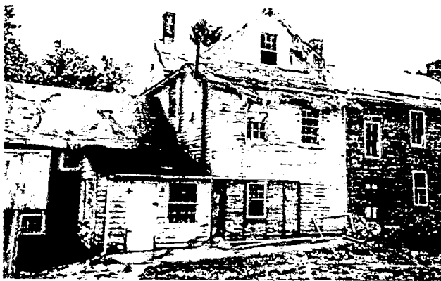
c.jpg Section of House to be Demolished Includes the one-story space and the two-story space immediately to its right. Both spaces have flat roofs that slope toward the photographer. Windows will be saved.
