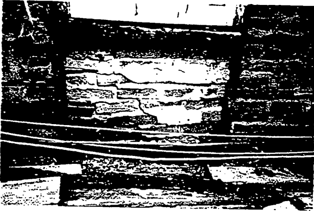
Detail of Structural problems. Foundation is crumbling.
