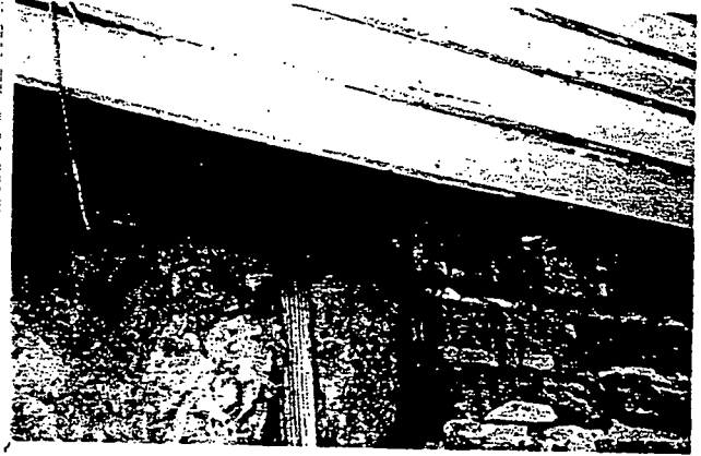
Detail of Structural Problems. Lintel is rotted away.
