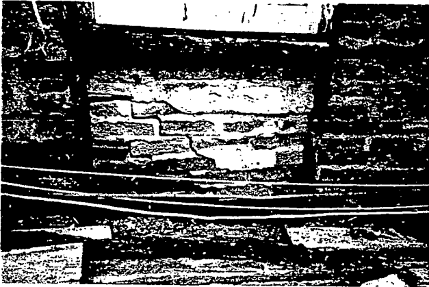
Detail of Structural problems. Foundation is crumbling.
