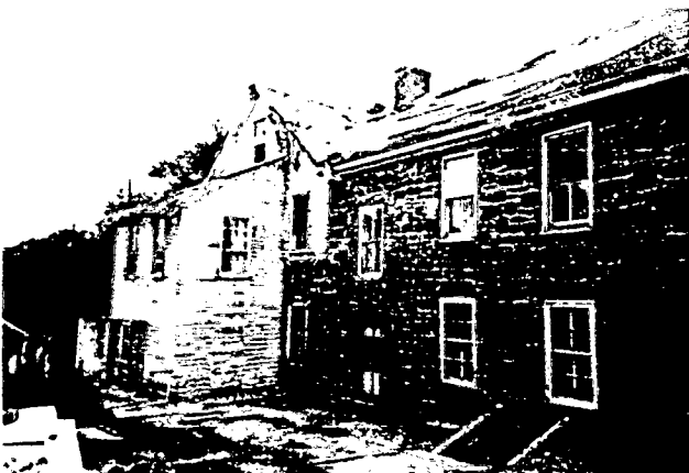
e.jpg South/West Elevation Section to be demolished has flat roof. Window will be saved.
