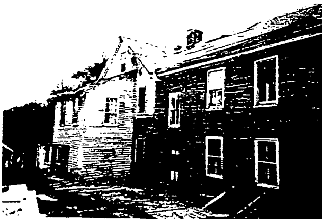
e.jpg South/West Elevation Section to be demolished has flat roof. Window will be saved.
