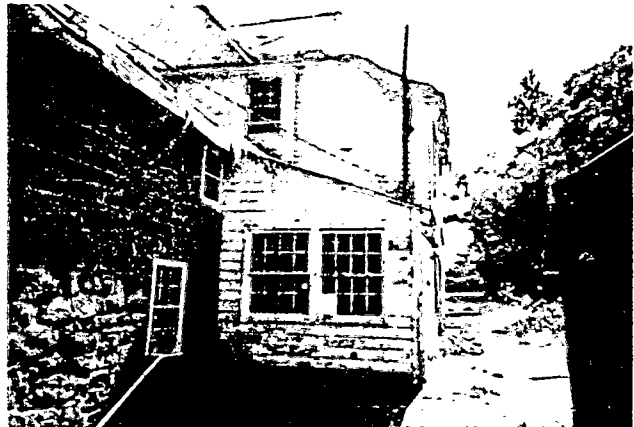
d.jpg North Elevation of Section to be Demolished Windows will be saved.
