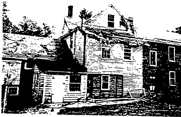
c.jpg Section of House to be Demolished Includes the one-story space and the two-story space immediately to its right. Both spaces have flat roofs that slope toward the photographer. Windows will be saved.
