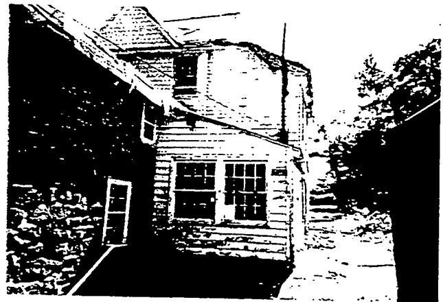
d.jpg North Elevation of Section to be Demolished Windows will be saved.
