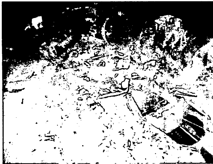
Figure 6: Deteriorated wearing surface from roof leaks
