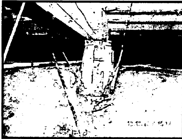
Figure 22. Wooden barrel that was used as the form for pouring the concrete footing for the center girder in the crawl space.
