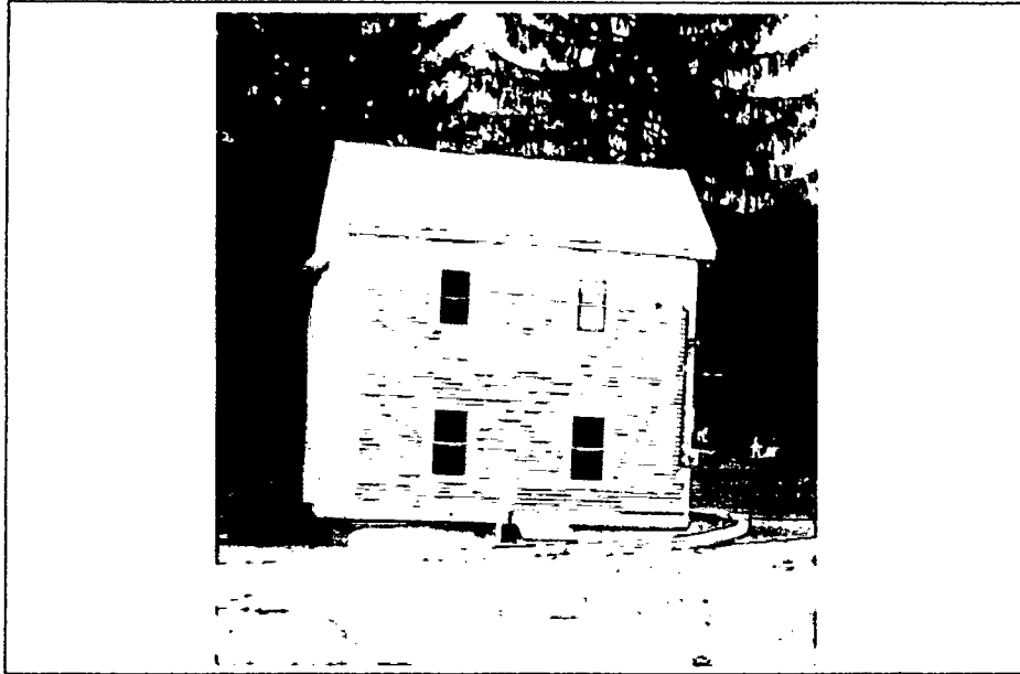
Detail: VIEW LOOKING NORTH (REAR VIEW)
