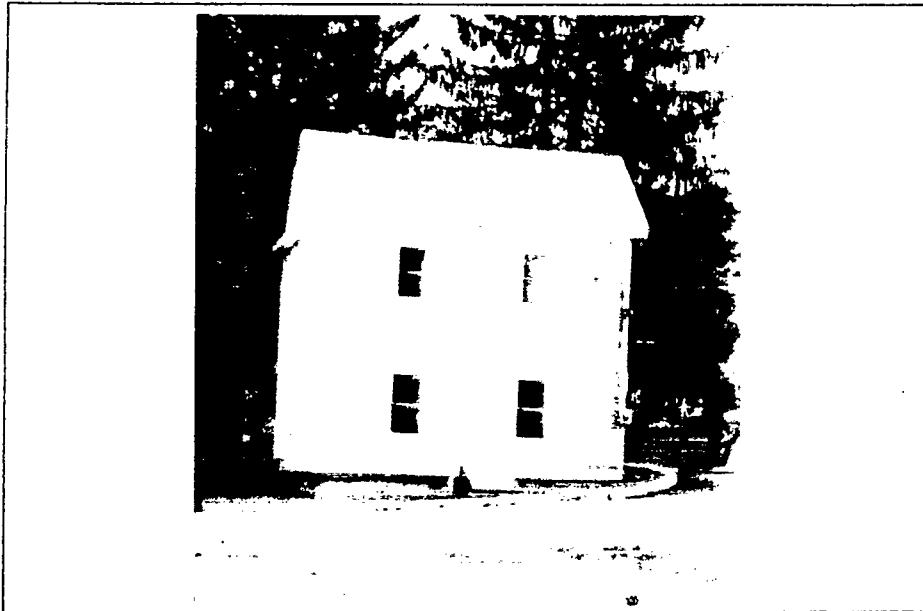
Detail: VIEW LOOKING NORTH (REAR VIEW)
