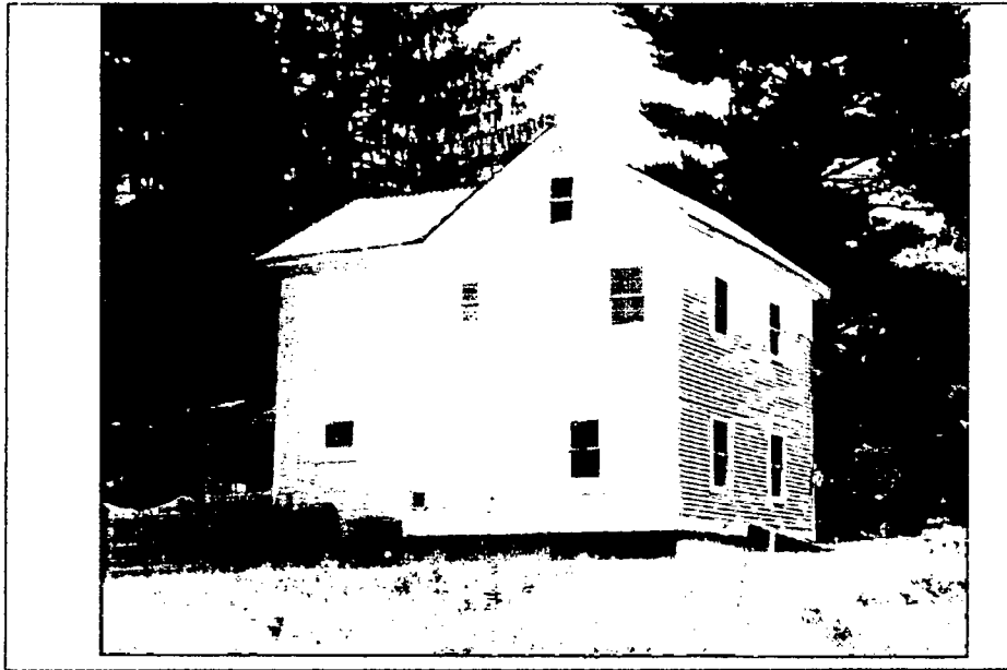
Detail: VIEW LOOKING EAST (RIGHT SIDE VIEW)
