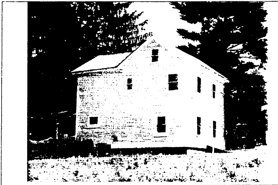
Detail: VIEW LOOKING EAST (RIGHT SIDE VIEW)
