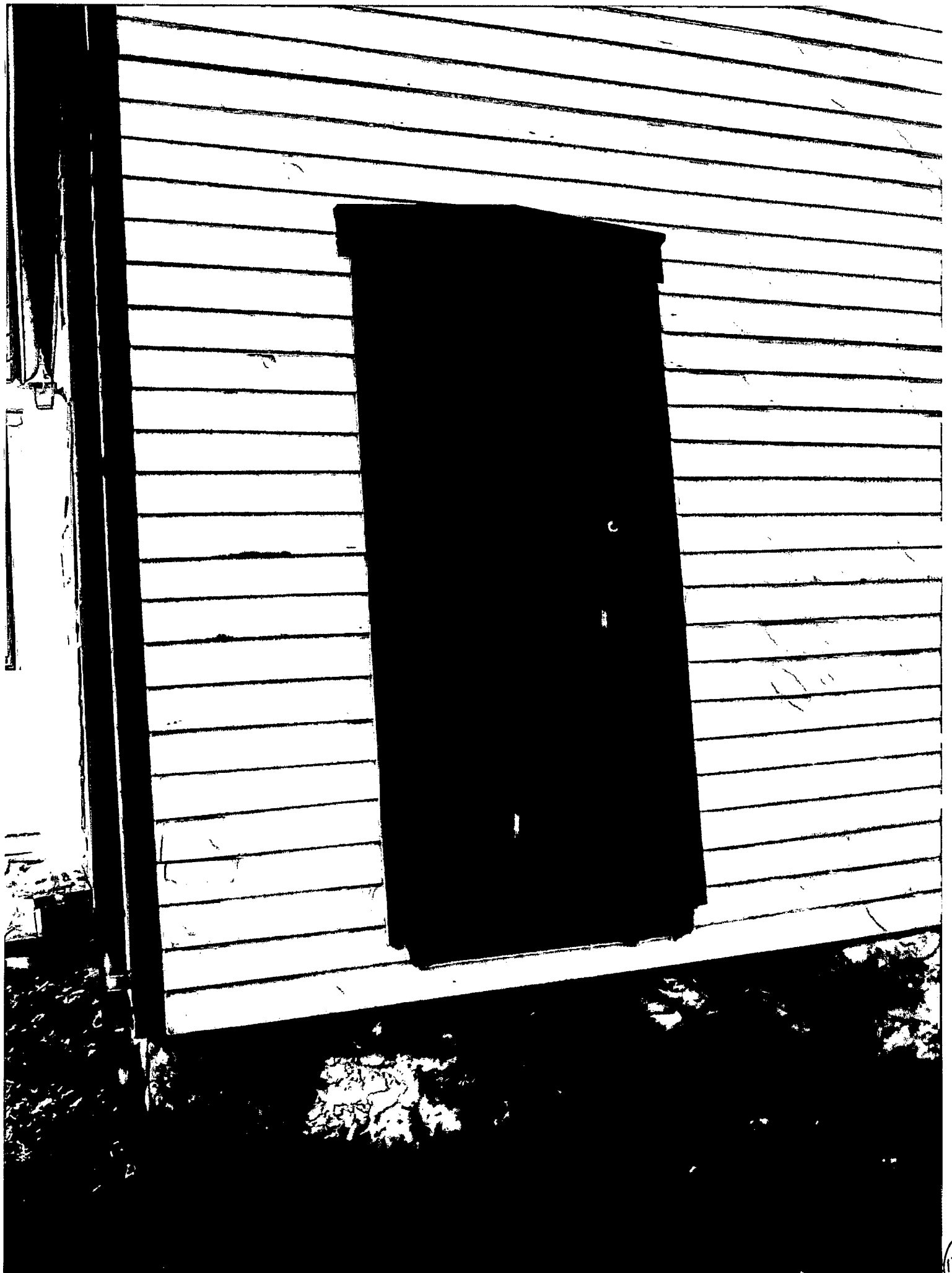
Side door showing need for stoop
