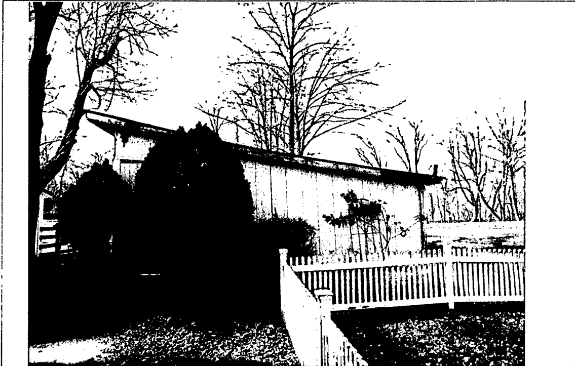
Detail: View of east elevation.
