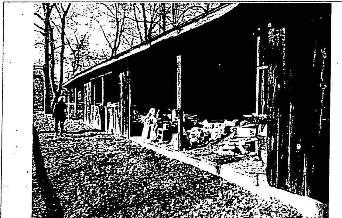
Detail: View of south elevation, looking west.
