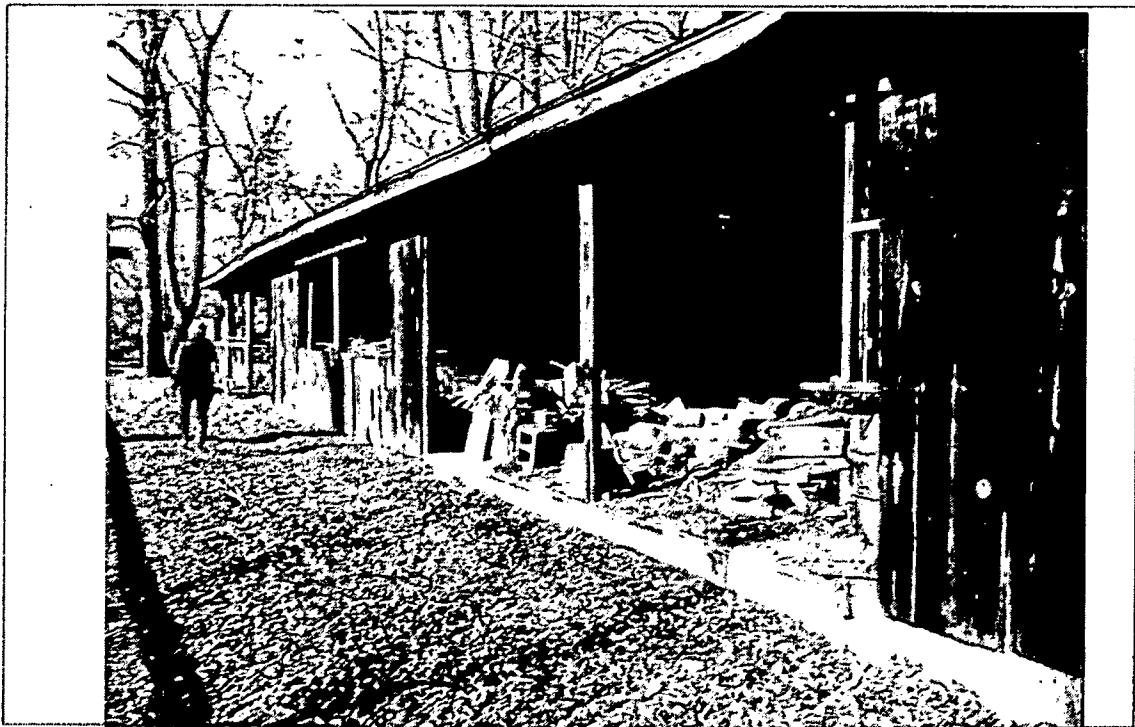
Detail: View of south elevation, looking west.
