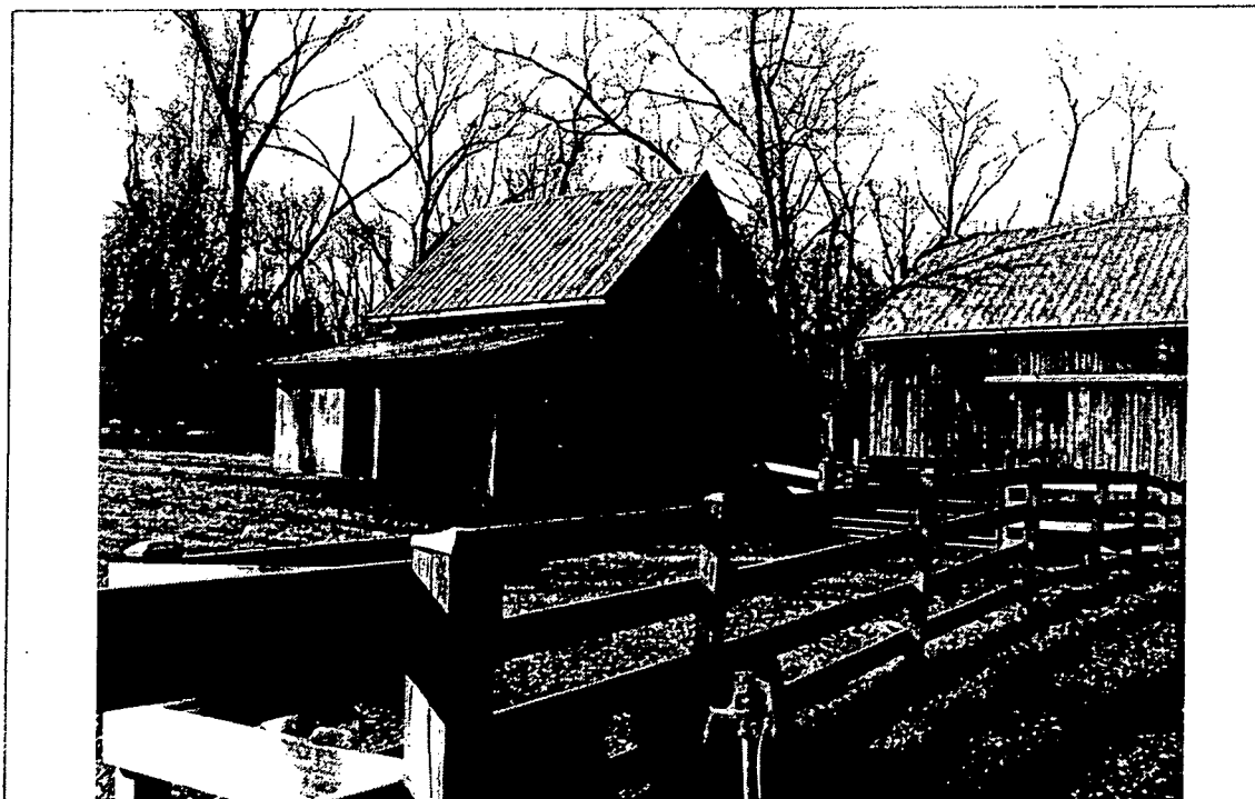
Detail: View of barns.
