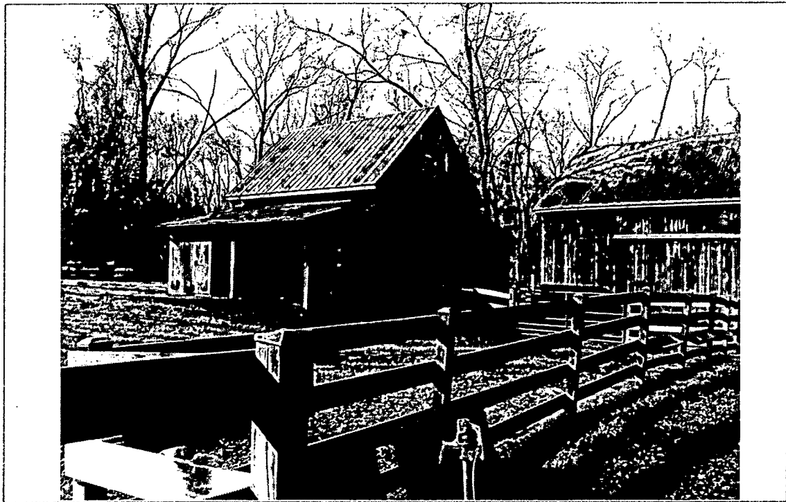
Detail: View of barns.
