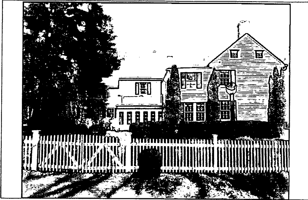
Detail: View of manor house.
