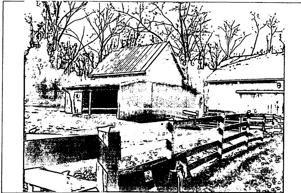
Detail: View of barns.
