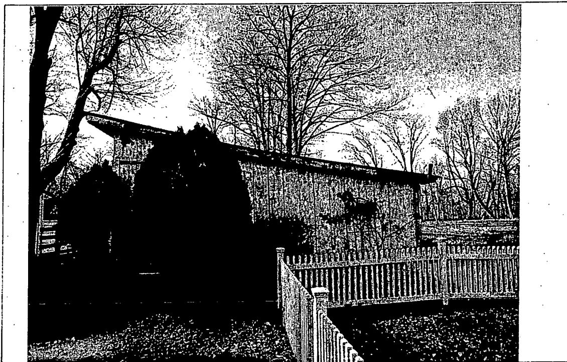
Detail: View of east elevation.
