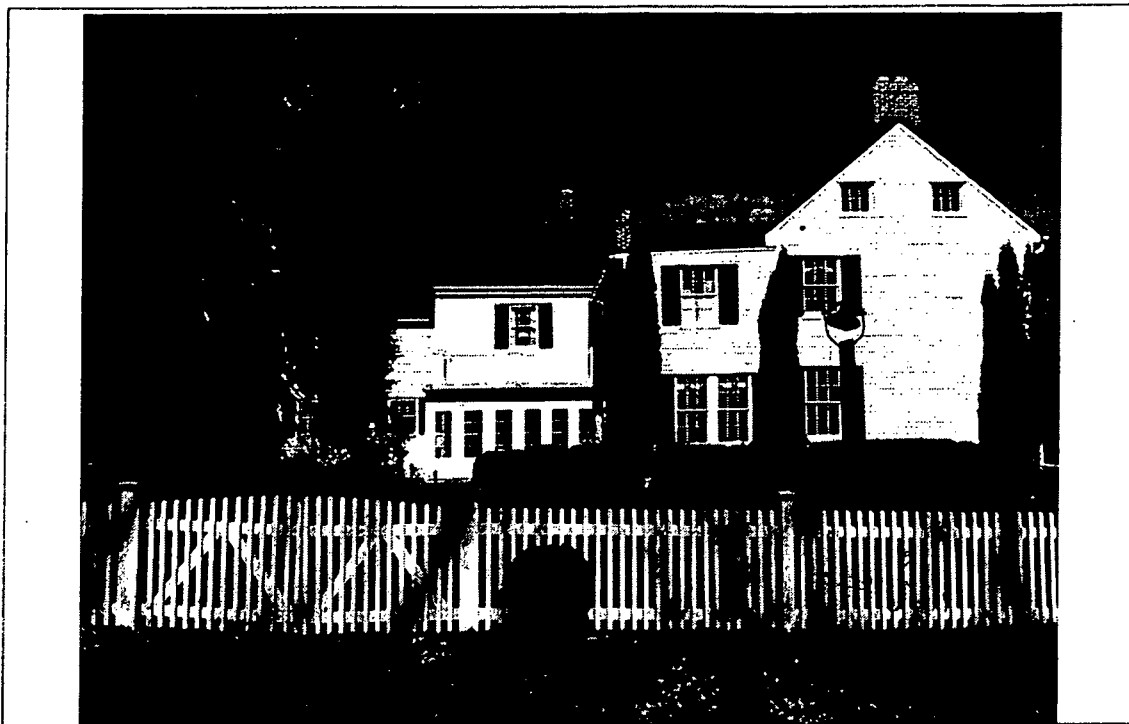
Detail: View of manor house.
