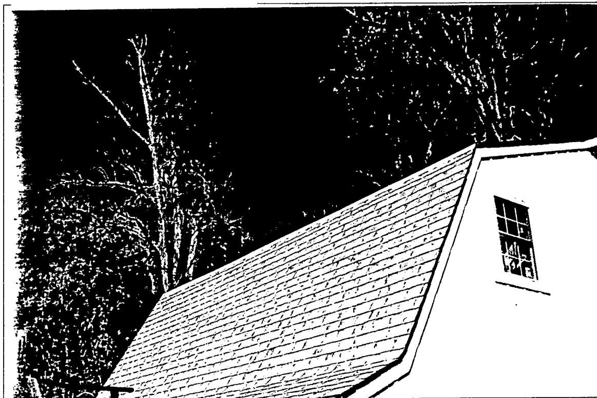
Detail: CLOSE UP OF ROOF
