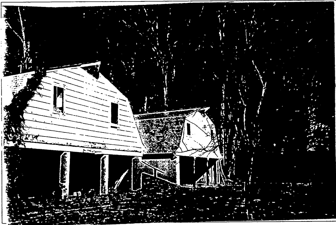
Detail: SOUTH FACING ROOF WHERE SOLAR PROPOSED
