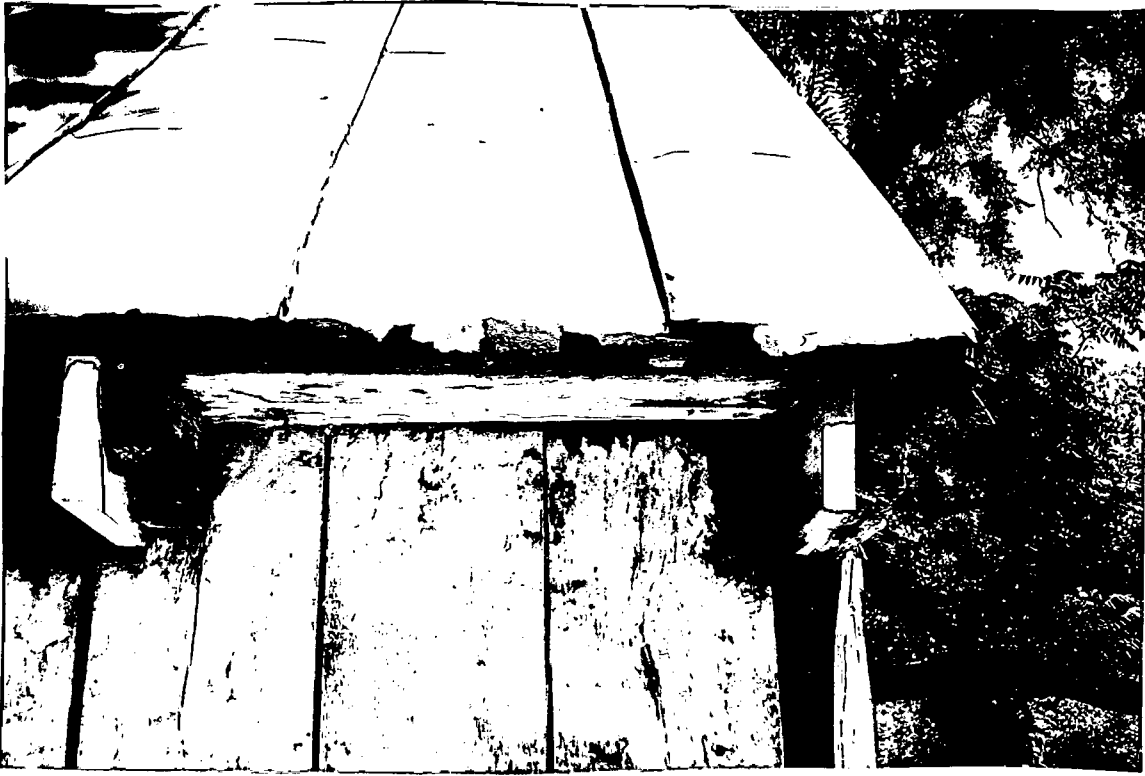
South side showing deteriorated overhang
