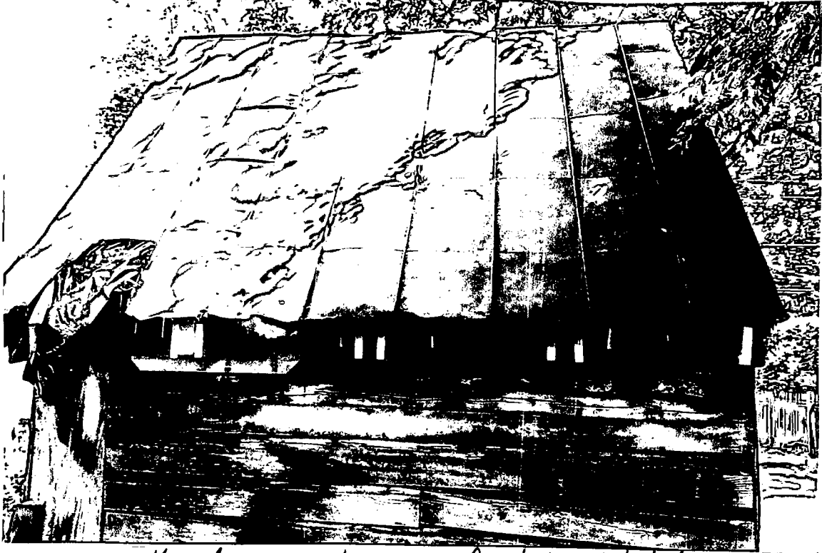
Detail: north side smokehouse roof - dilapidated terne
