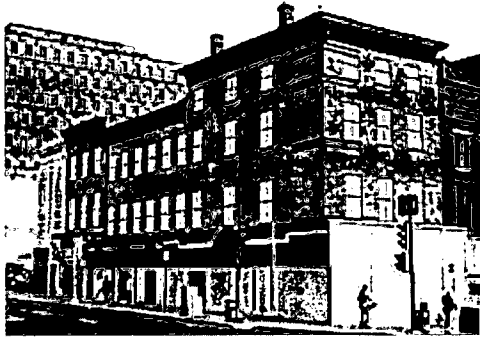
Urban buildings awaiting rehabilitation often need additional protection from unwanted entry and graffiti. This commercial building uses painted plywood panels to cover its glass storefronts. The upper windows on the street sides have been painted to resemble 19th century sash. Photo: NPS files.
