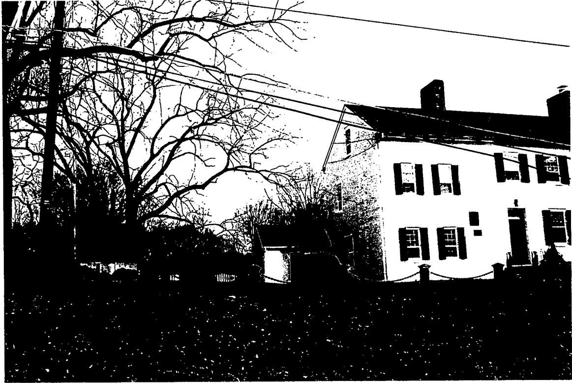
DETAIL: 205 MARKET ST. BROOKVILLE SOUTH VIEW SHOWING SMOKEHOUSE & PANTRY ADDITION
