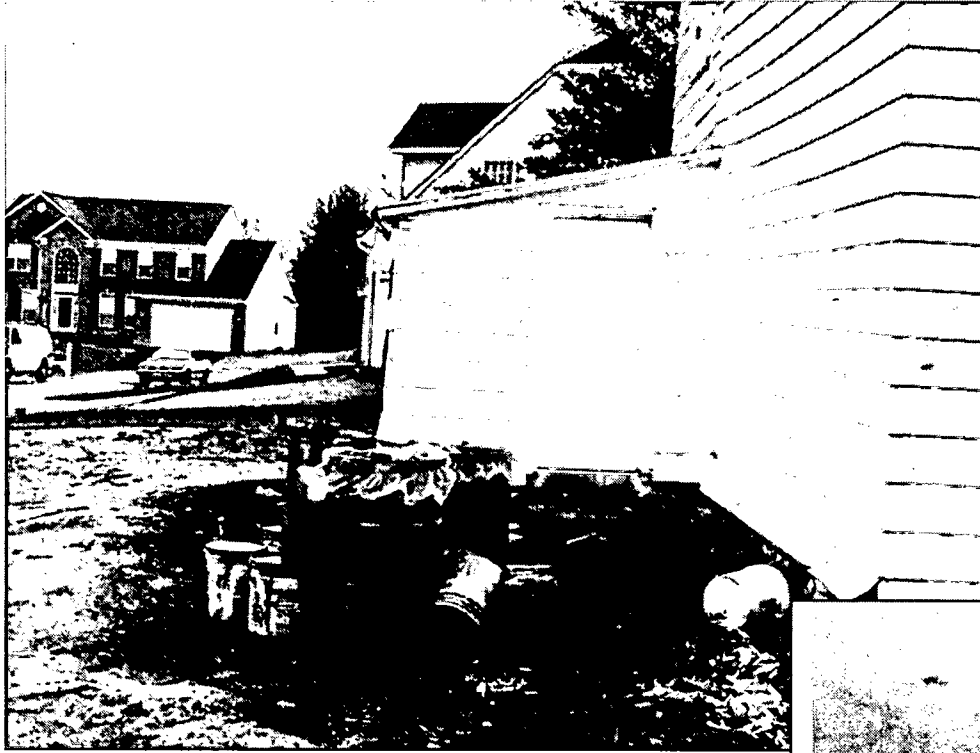
Existing She Roof Addition - exterior
