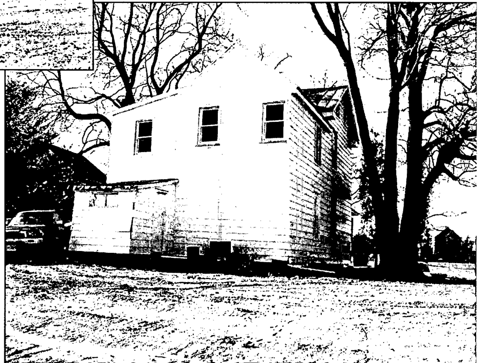
Left Side (northeast) Elevation
