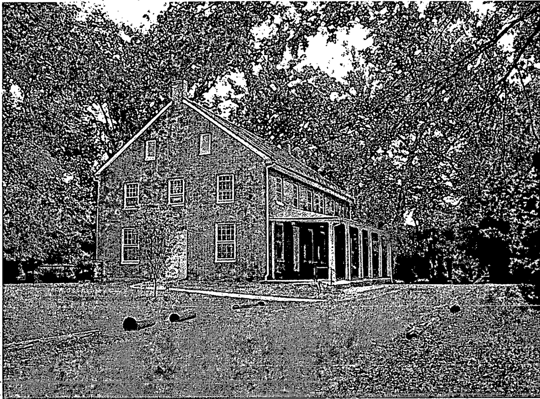
The historic Meeting House and rural road viewed from the northeast. The Meeting House will be untouched by the proposed project.
