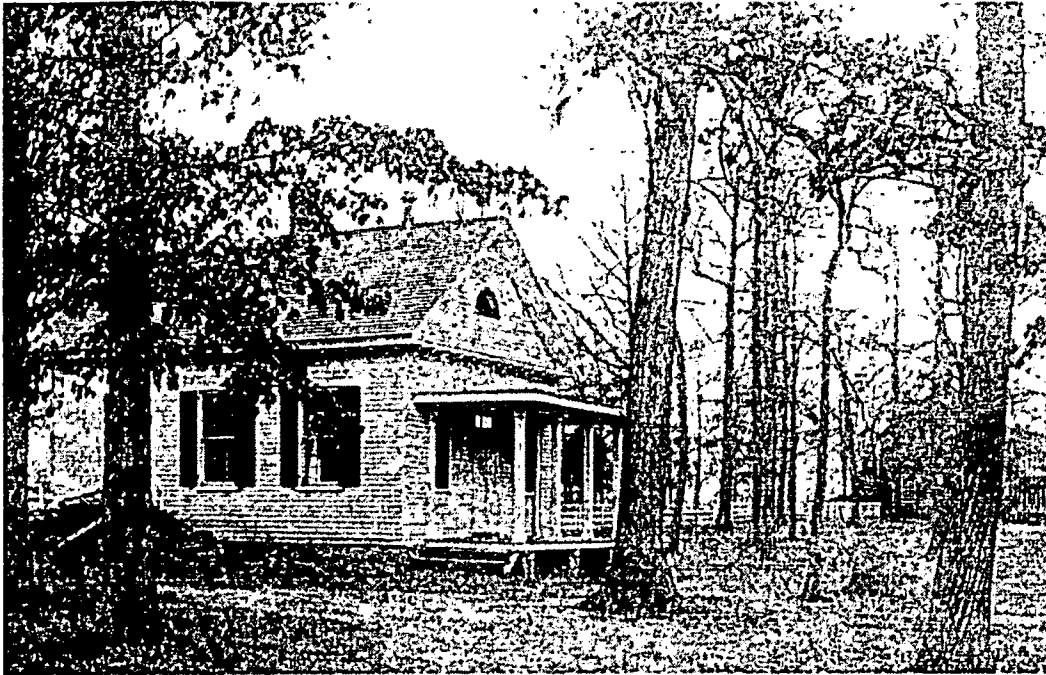
Historic photo of the Lyceum taken from the northwest. The meeting house is visible to the south. If the original lap siding is intact, it will be restored.
