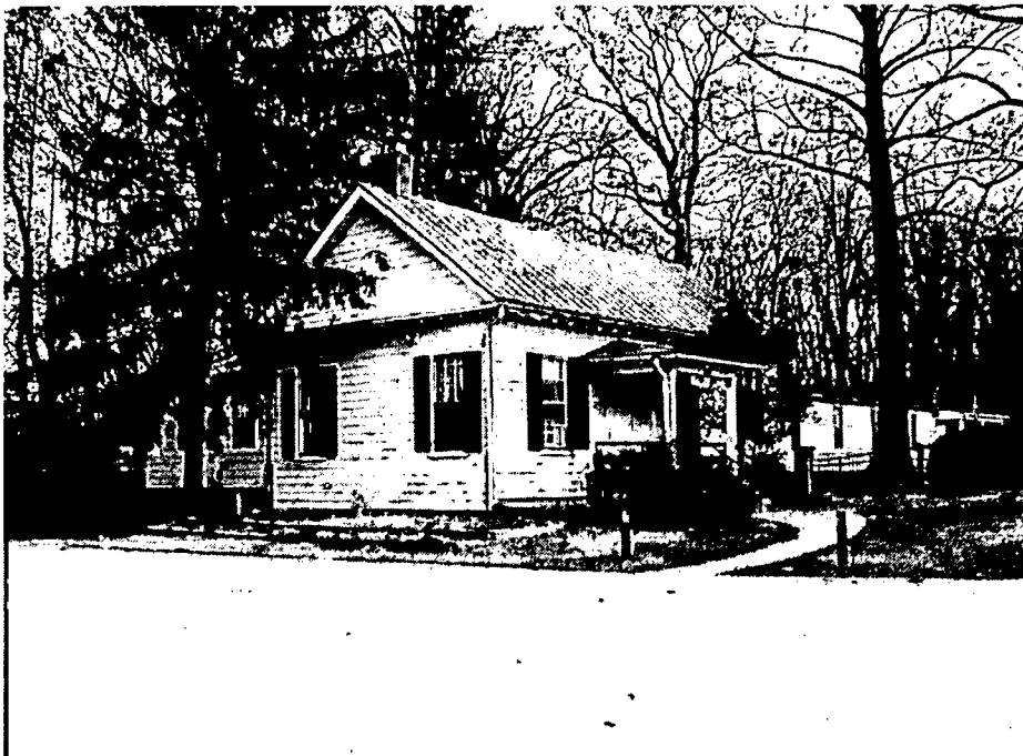
Current view of the Community House from the southwest parking lot showing south and west facades. The recessed east wing of the building visible in the photo will be demolished (built 1978 and 1985). The back low-slope addition on the north side will remain. The visible corner of the graveyard fence will be chamfered (Two stone fence posts will replace the one.) The tulip poplar will be removed.
