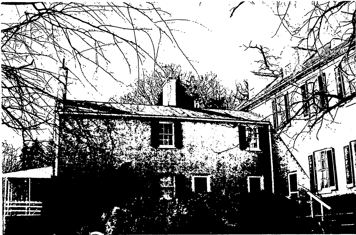
812 Lindsey Manor Lane – TOP: view of East-facing wing. BOTTOM: Close up of 3 dormers and roof of South-facing side of house
