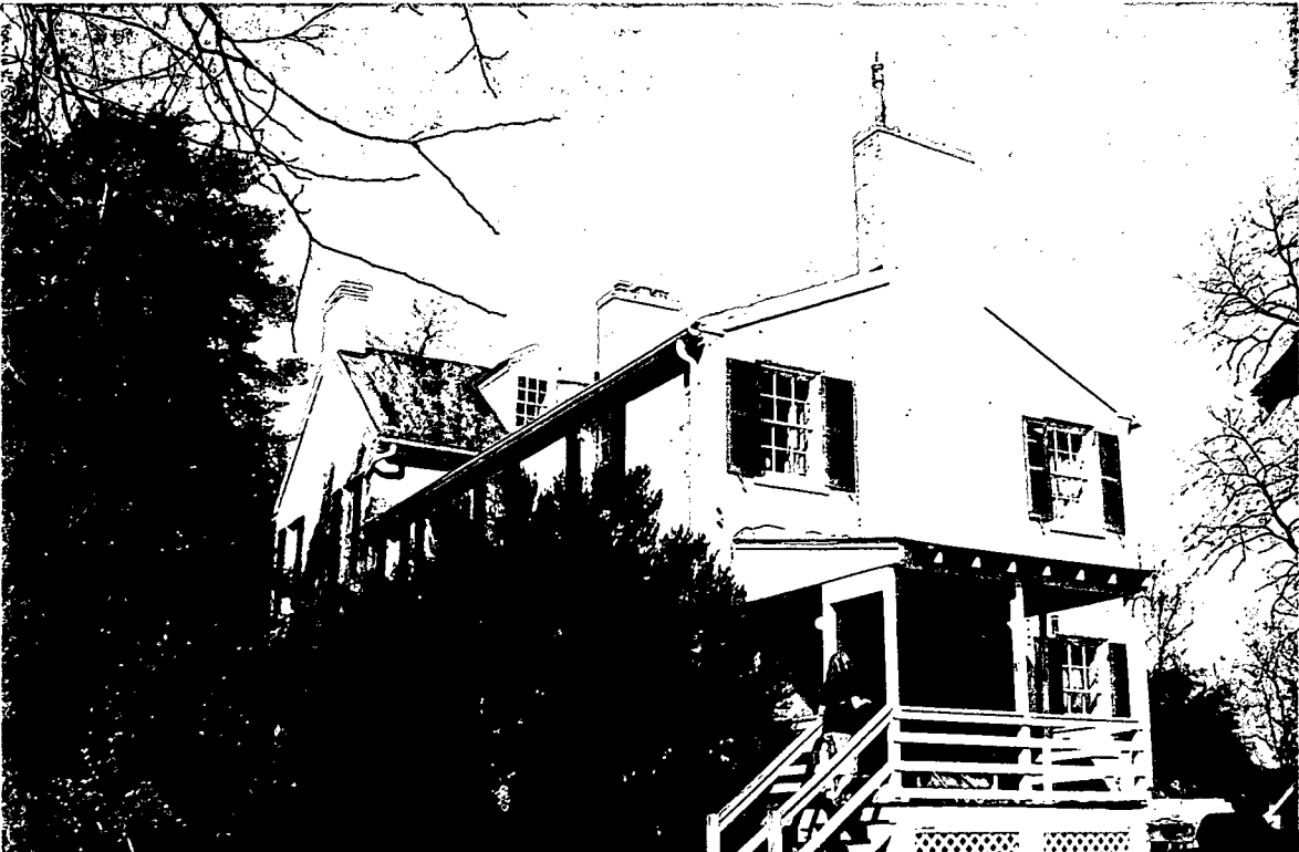
(bottom) 812 Lindsey Manor Lane – Rear porch of the wing and West-facing side. Roof of the Manor House and one dormer is visible in back.
