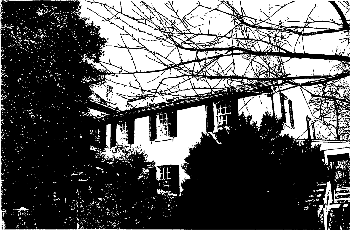
(top) 812 Lindsey Manor Lane – West-facing side of the wing
