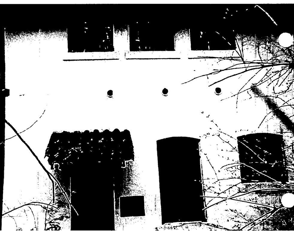
Existing Rear Elevation (facing home from street)
