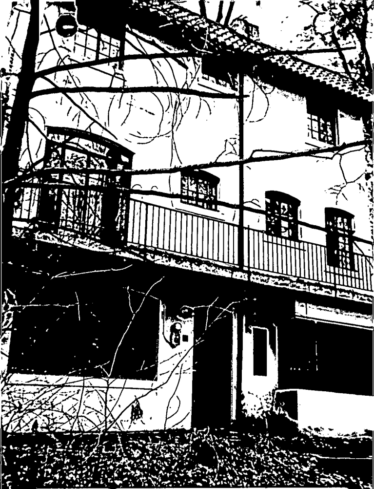
Existing Right Elevation. (facing home from street)
