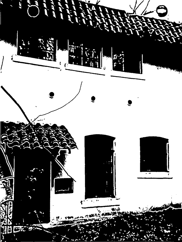
Existing Rear Elevation (facing home from street)
