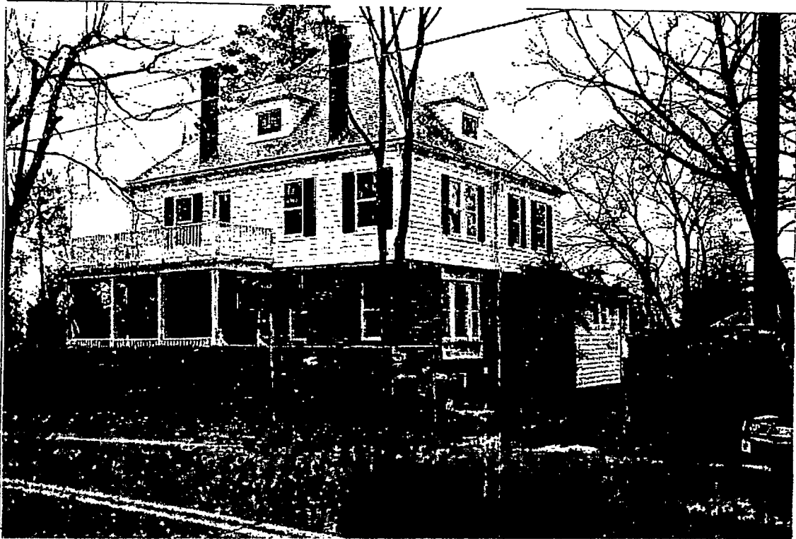
Detail: REAR OF HOUSE FROM STONEY BROOK
