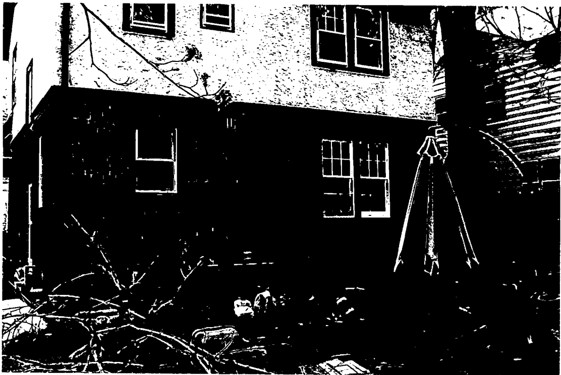
Detail: Back of home prior to construction
