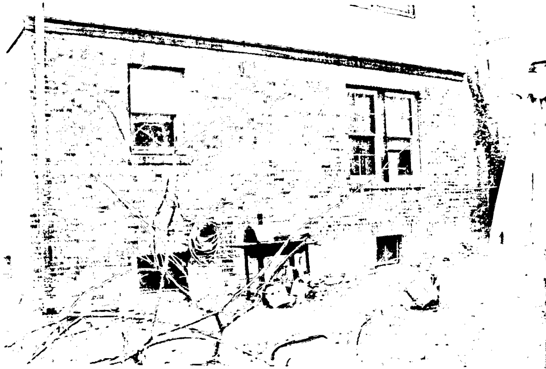
Detail: Back of home prior to construction
