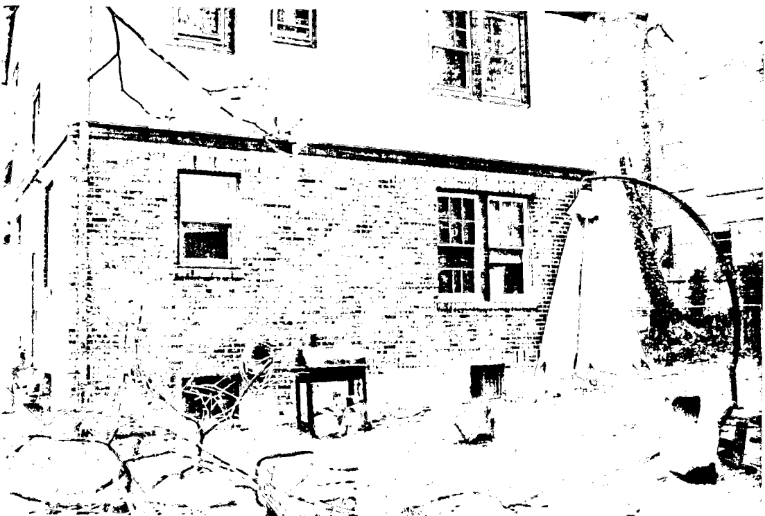
Detail: Back of home prior to construction
