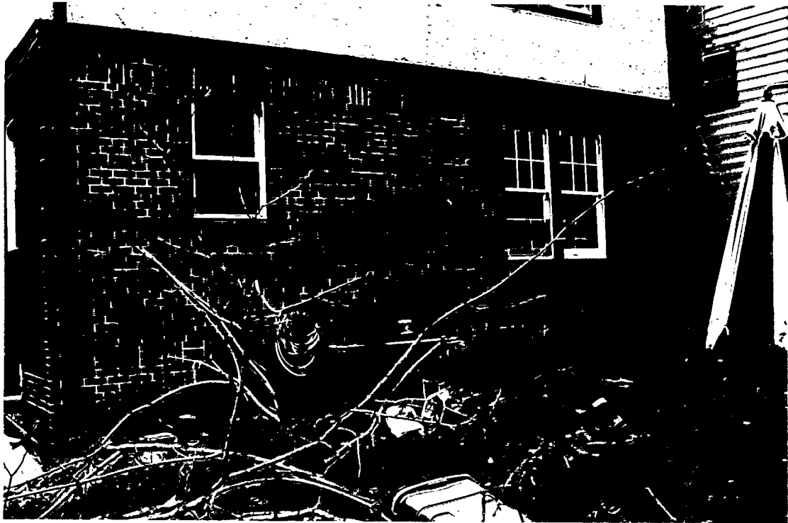
Detail: Back of home prior to construction
