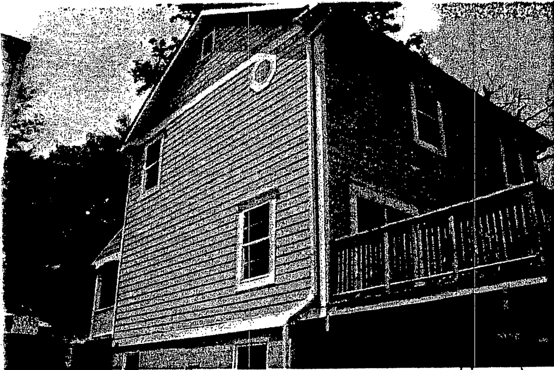
RIGHT/SOUTH ELEVATION (FROM REAR OF HOUSE), SUBJECT PROPERTY
