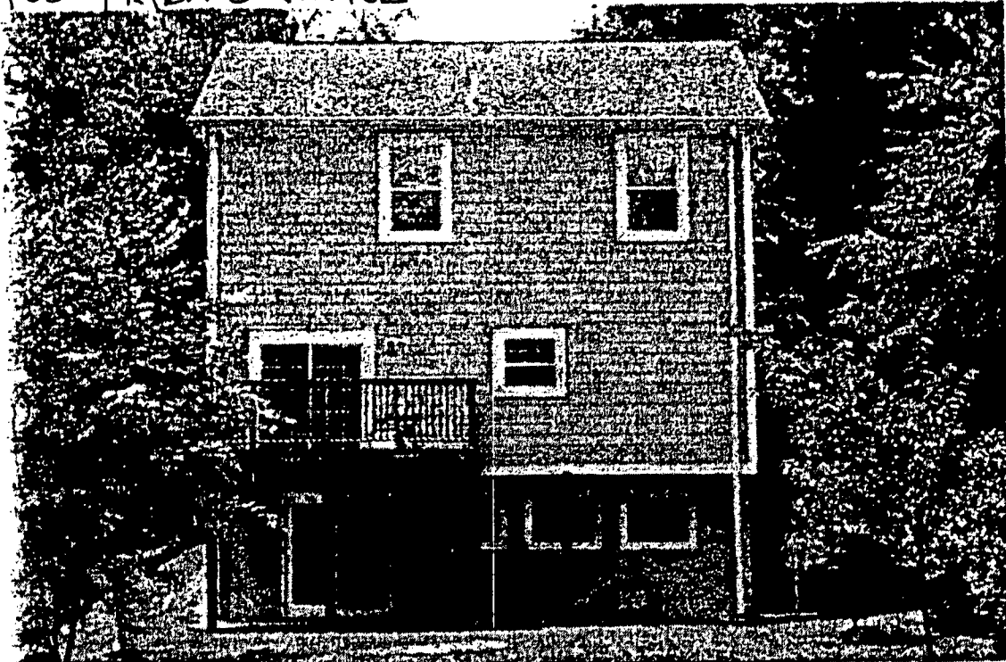
REAR/EAST ELEVATION, SUBJECT PROPERTY
