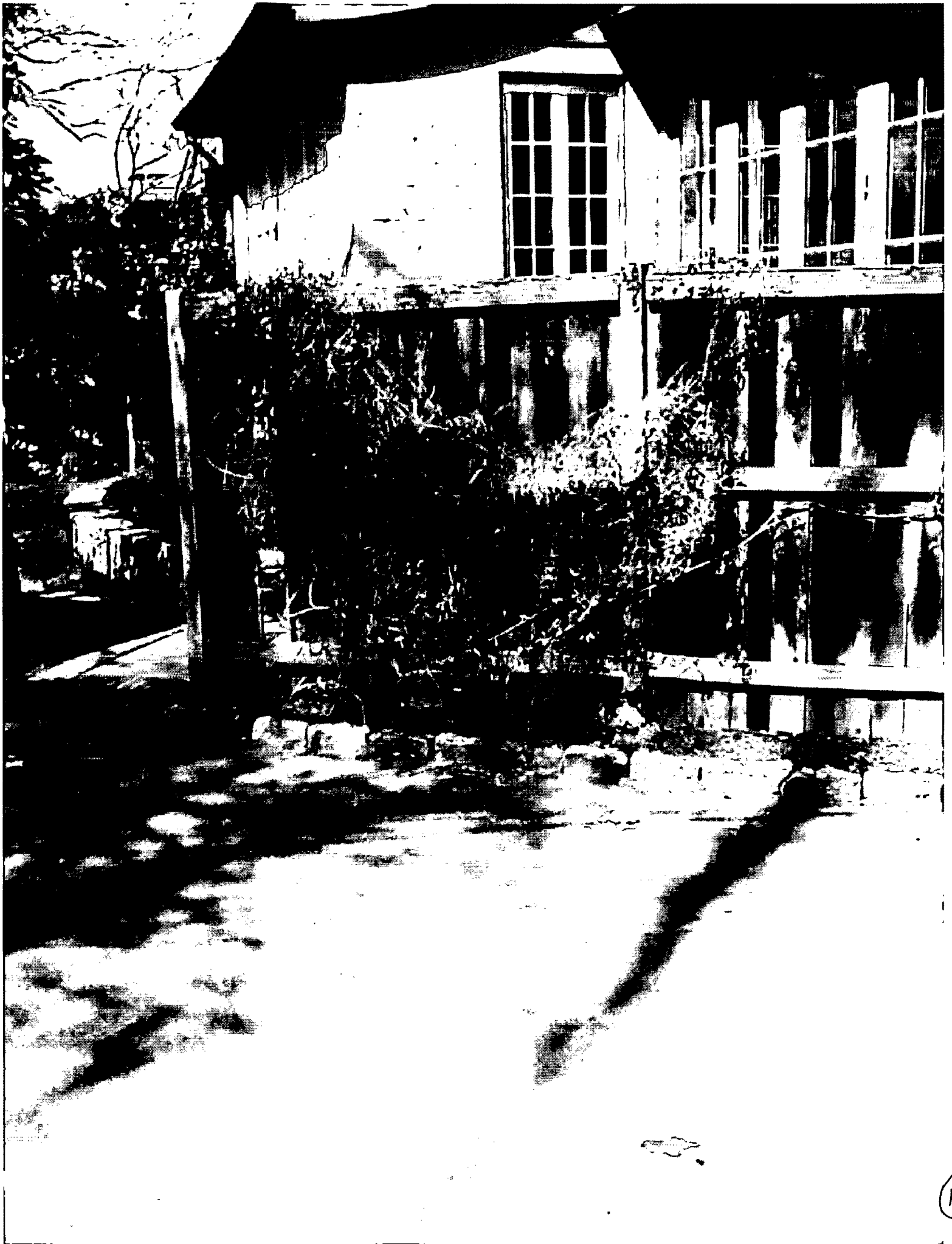
EXISTING FENCE LOOKING FROM NEIGHBORS ACROSS DRIVEWAY
