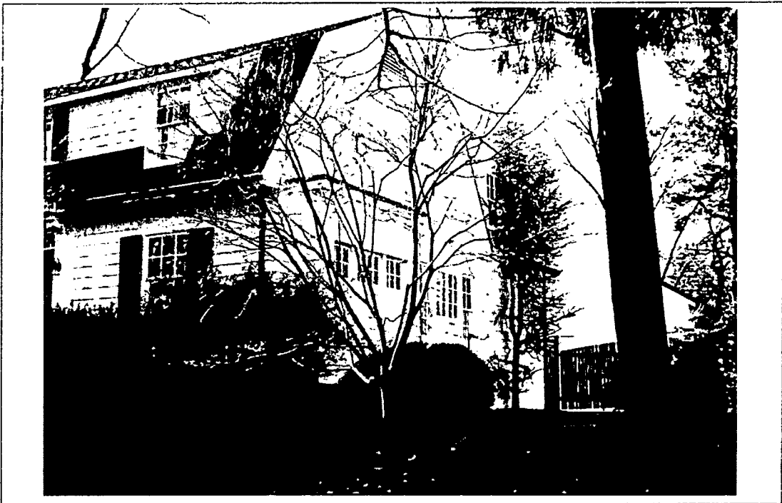
Detail: Right Side of House (2000 Rear Addition was stepped back from original structure)
