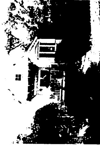
Rear Elevation A later addition is constructed on a brick foundation, exposure of the brick ranges from 30" to 40" in height.
