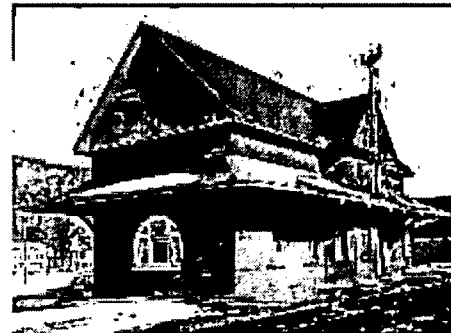
Gable and pent roof in excellent condition.
