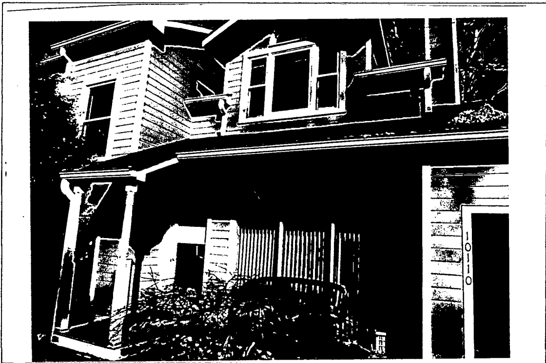
Detail: SOUTH FACADE
