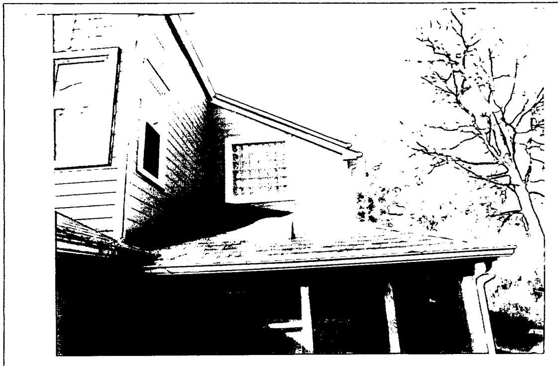
Detail: VIEW FROM NORTHEAST
