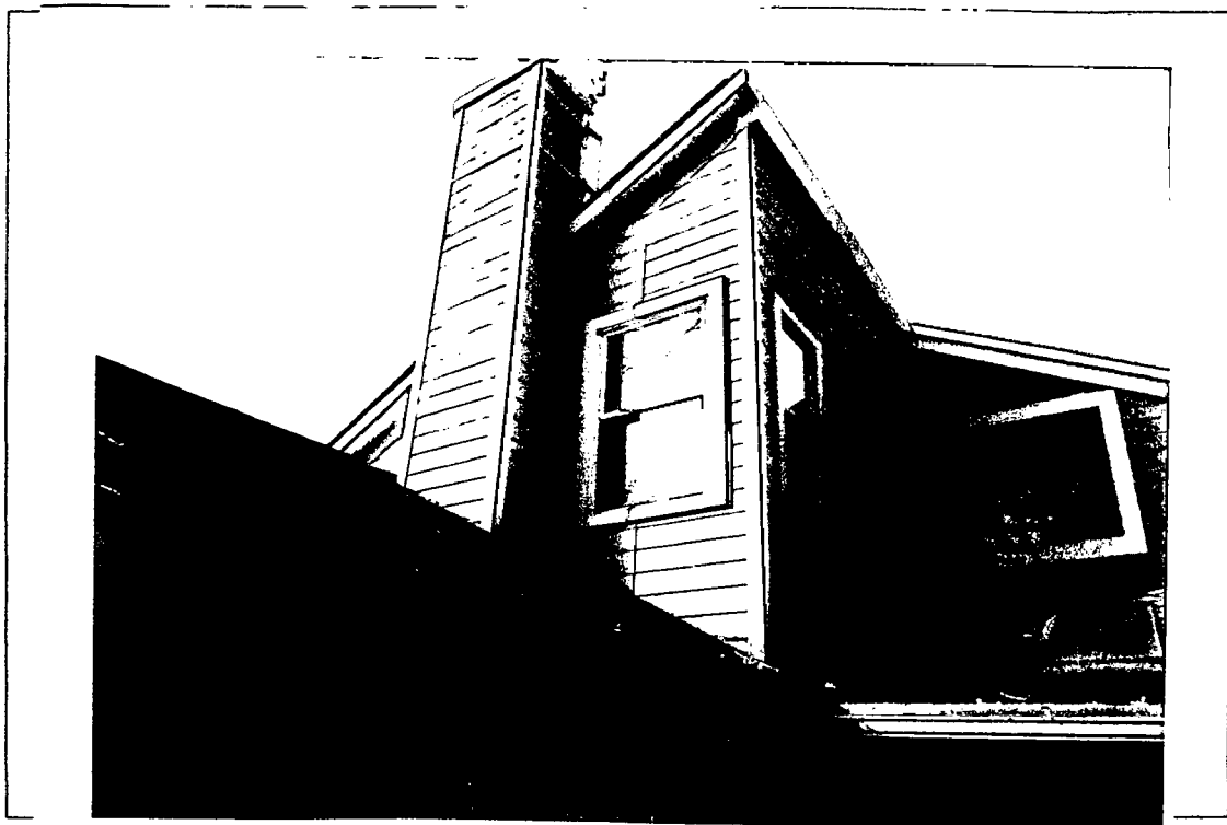
Detail: VIEW FROM NORTHEAST
