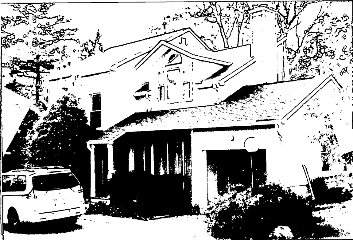
Detail: SOUTH FACADE FROM SOUTHEAST
