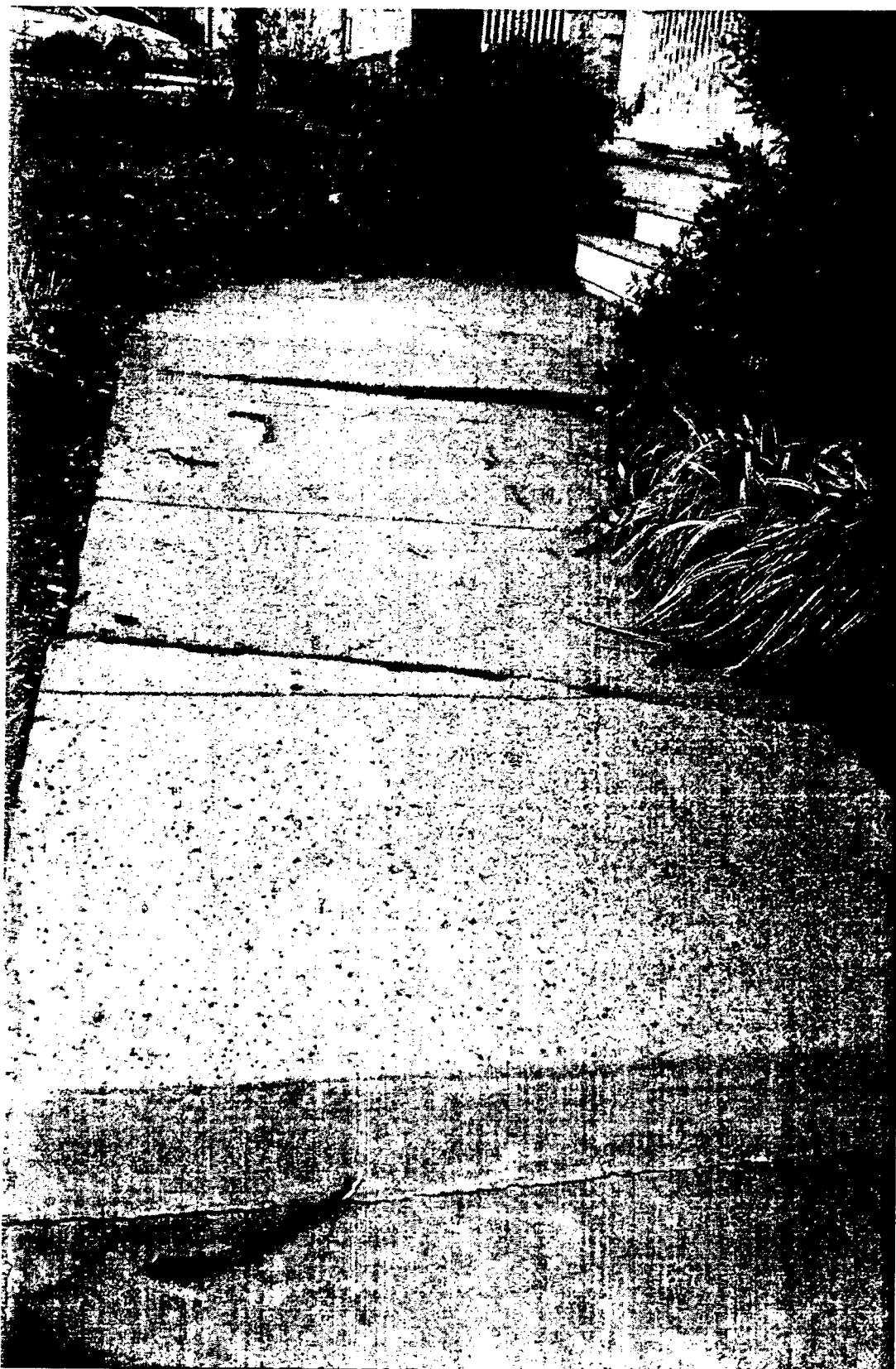
Front walk detail showing current condition and need for replacement.
