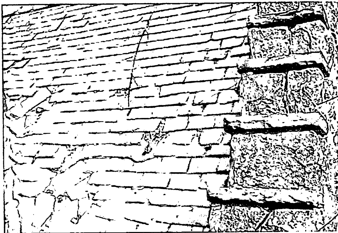
5415 Mohican Road, Bethesda Roof damage
