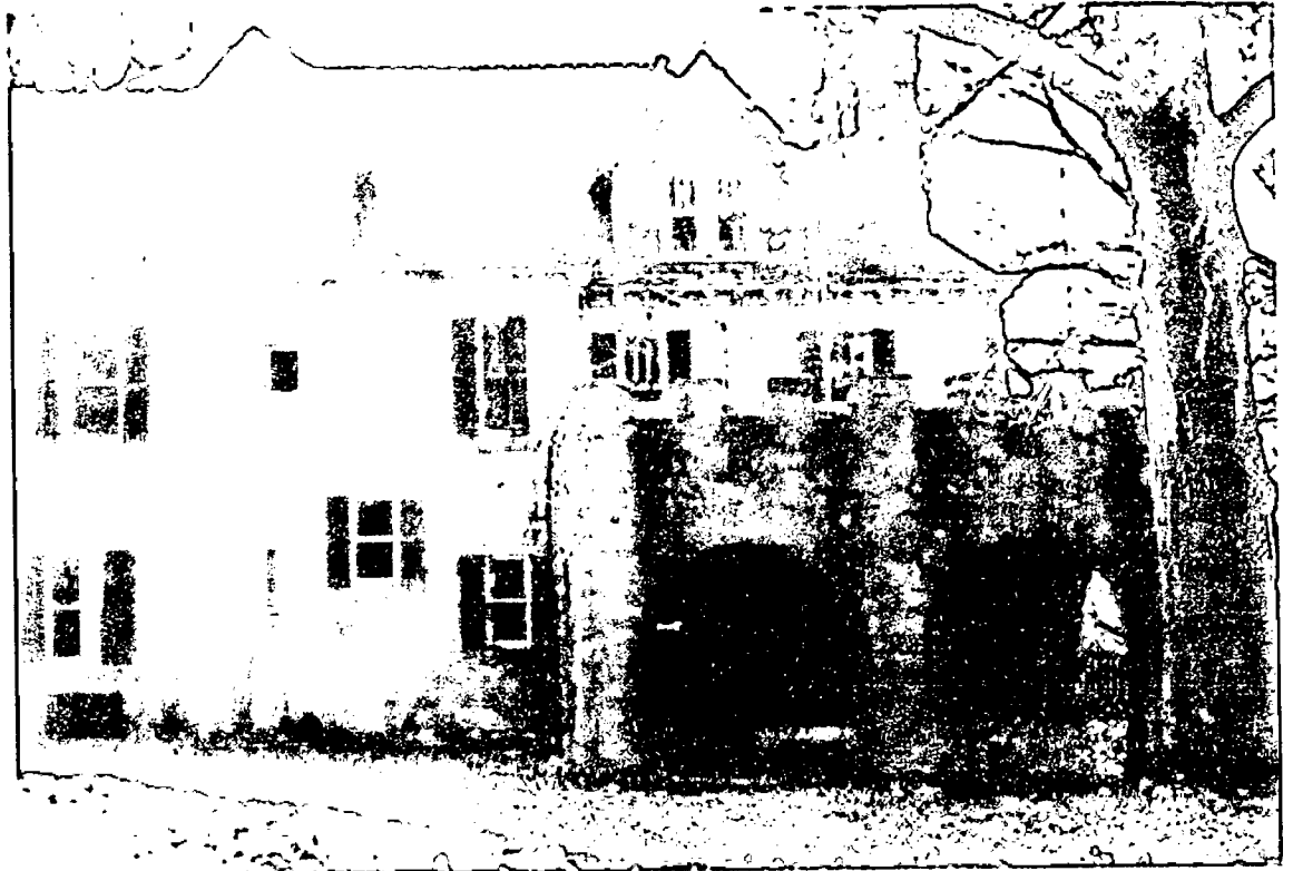
5415 Mohican Road, Bethesda North view
