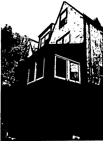
VIEW OF EXISTING REAR ADDITION FROM BOTTOM OF DRIVEWAY
