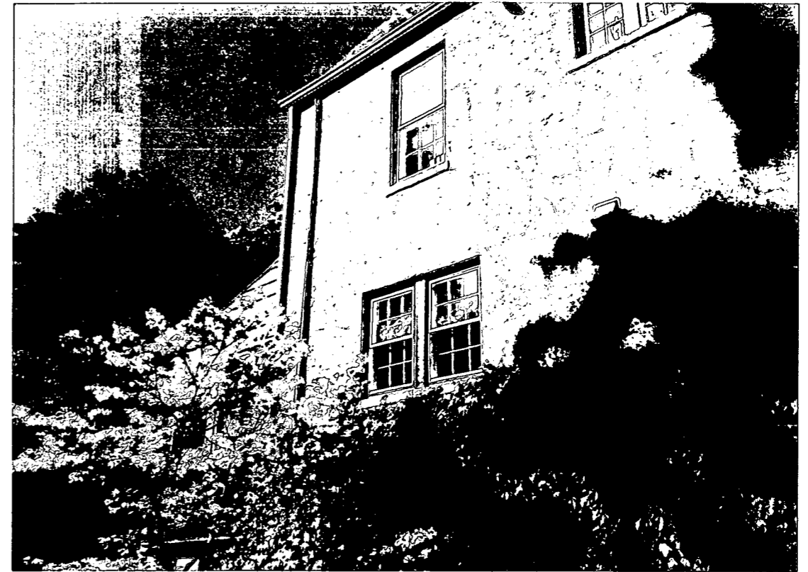
EXISTING SIDE ELEVATION VIEWED FROM DRIVEWAY
