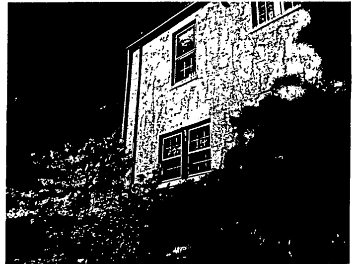
EXISTING SIDE ELEVATION VIEWED FROM DRIVEWAY
