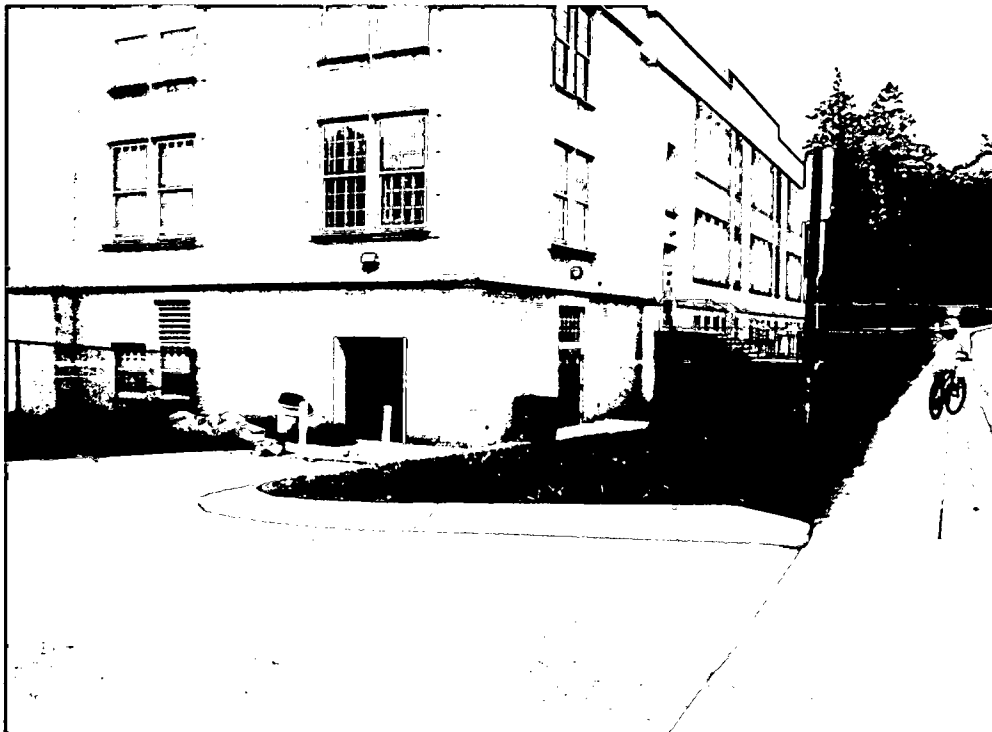
Detail: VIEW FROM HILLCREST PLACE FACING SOUTH TO PROPOSED LOCATION FOR DRIVEWAY GATE
