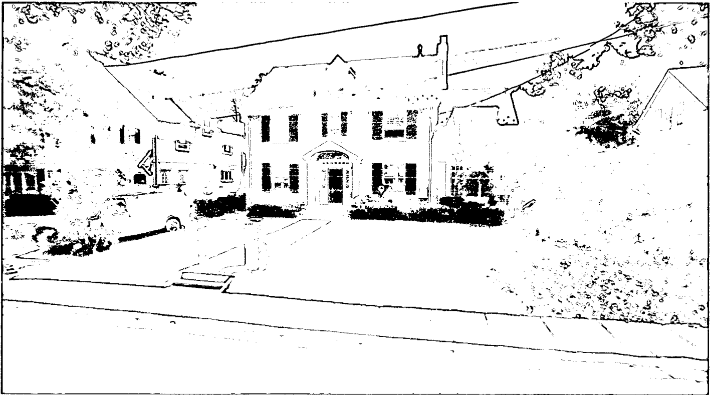
VIEW OF EXISTING FRONT FACADE FROM BRADLEY LANE
