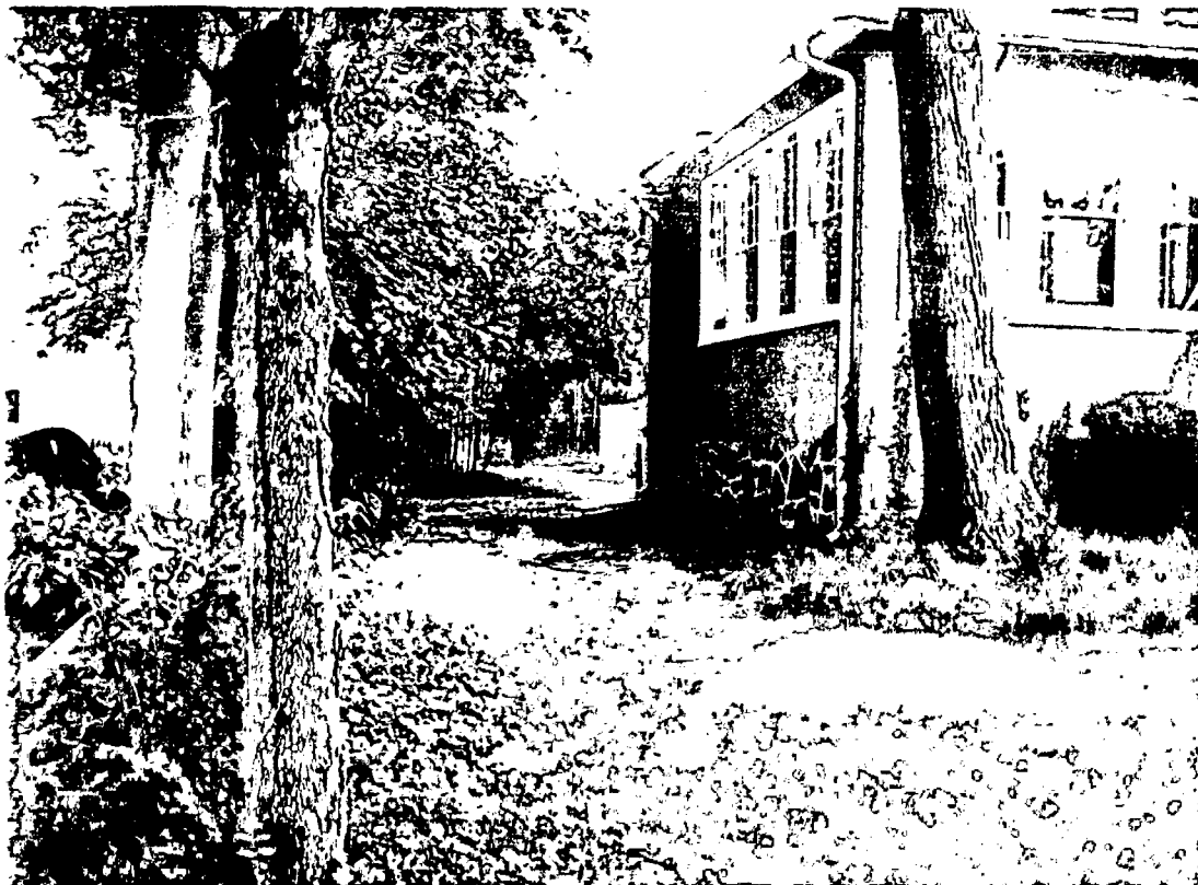
Senhauser Property, 3712 Bradley Lane East Side Yard View from Bradley Lane Proposed Skip Laurel Hedge and Gate Location
