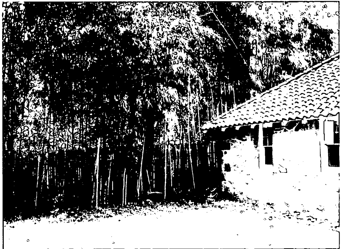
Rear Fence Line Looking West
