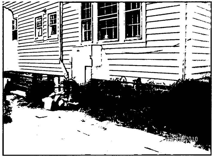
View of side of house where trash enclosure will be built
