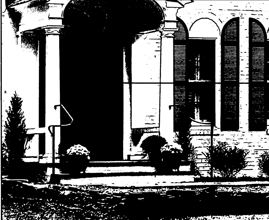
EXAMPLE OF WROUGHT IRON RAILING WITH SWEEP END AND LAMBS TONGUE. SIMILAR DETAILS TO THE PROPOSED RAILING.
