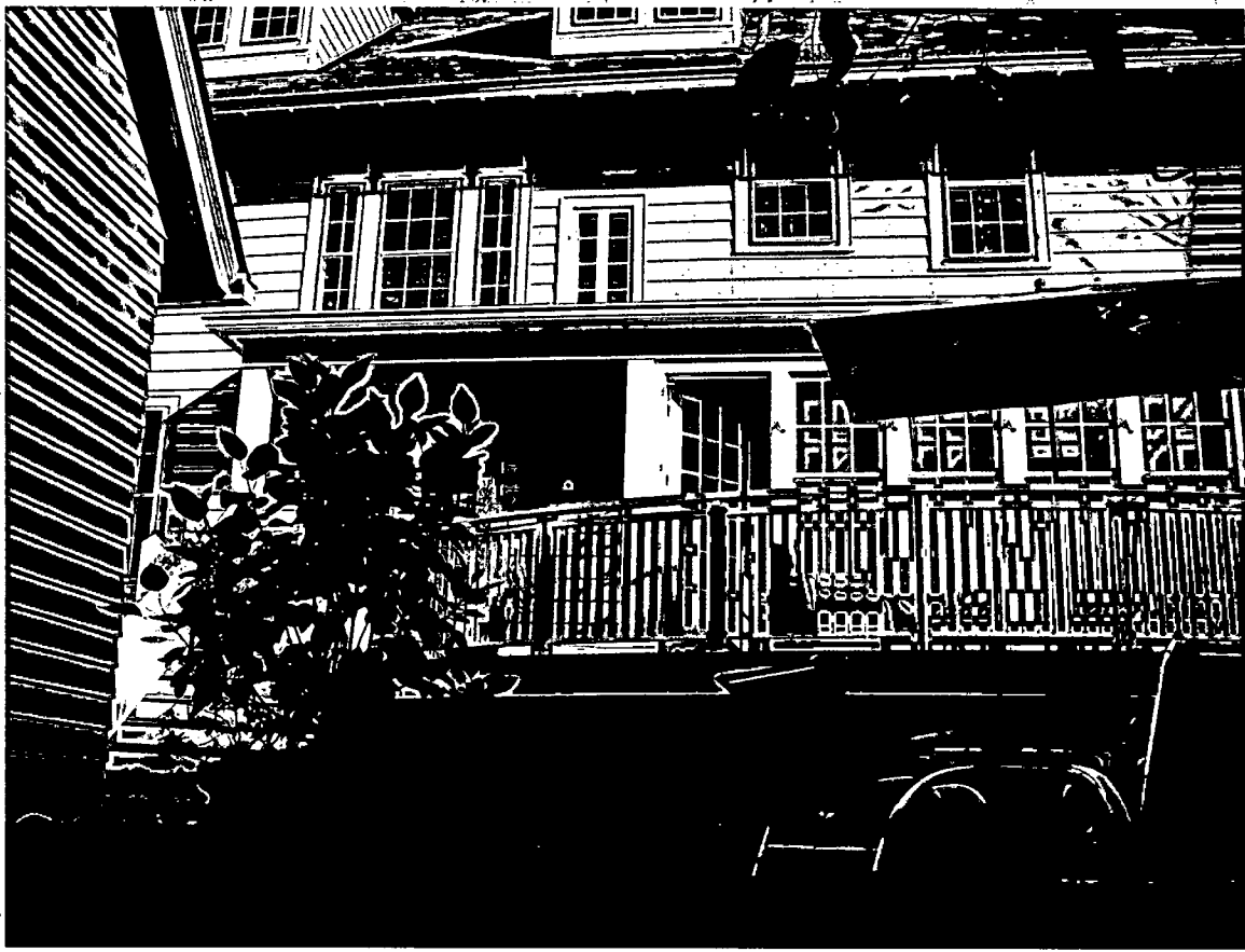
Back of house. Photo taken from back fence.
