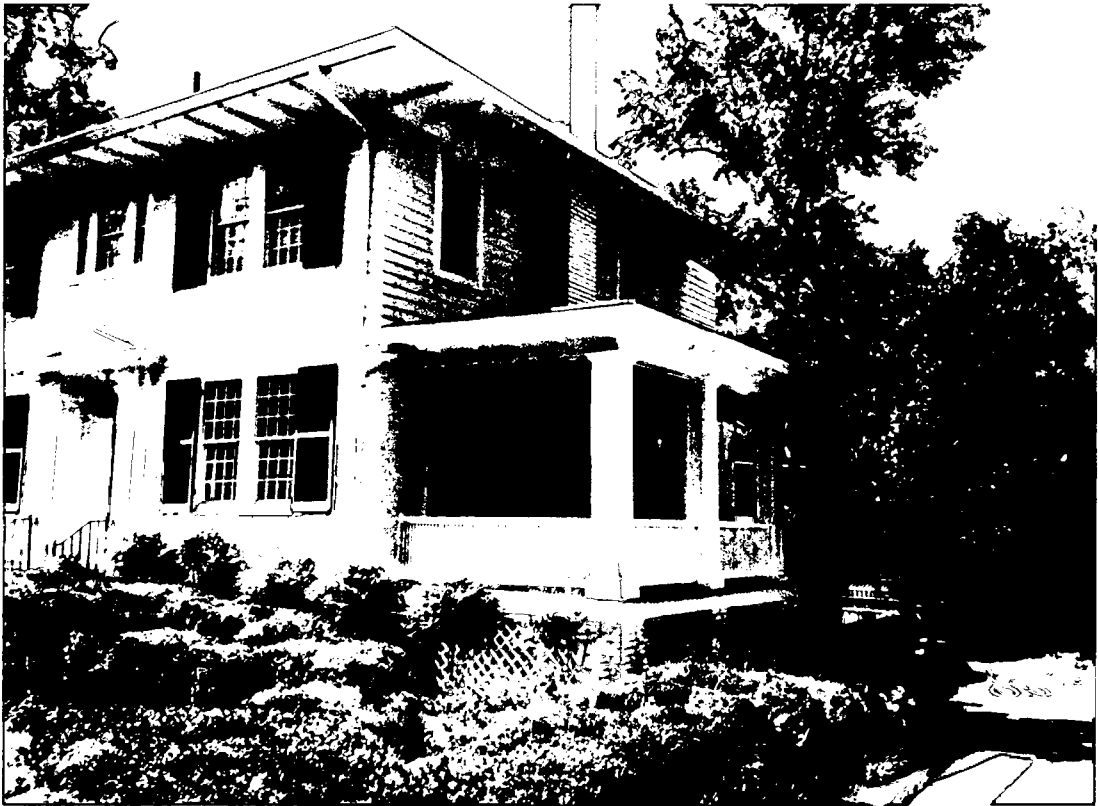
Existing Side Porch
