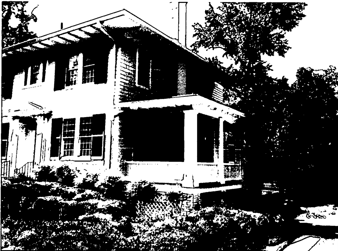
Existing Side Porch
