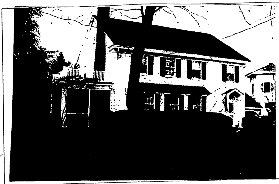
Detail: 19 Quincy St - side view from left
