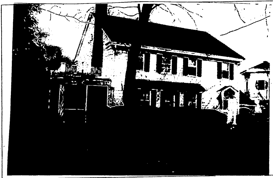
Detail: 19 Quincy St - side view from left
