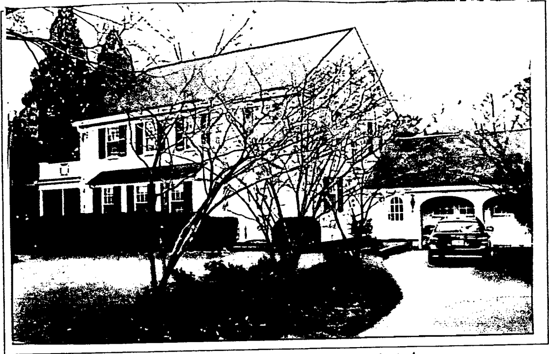
Detail: 19 Quincy St - side view from right - garage on right
