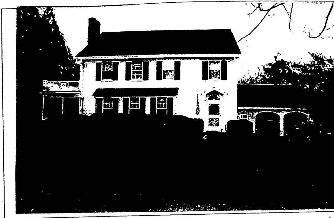
Detail: 19 Quincy St - front view from street
