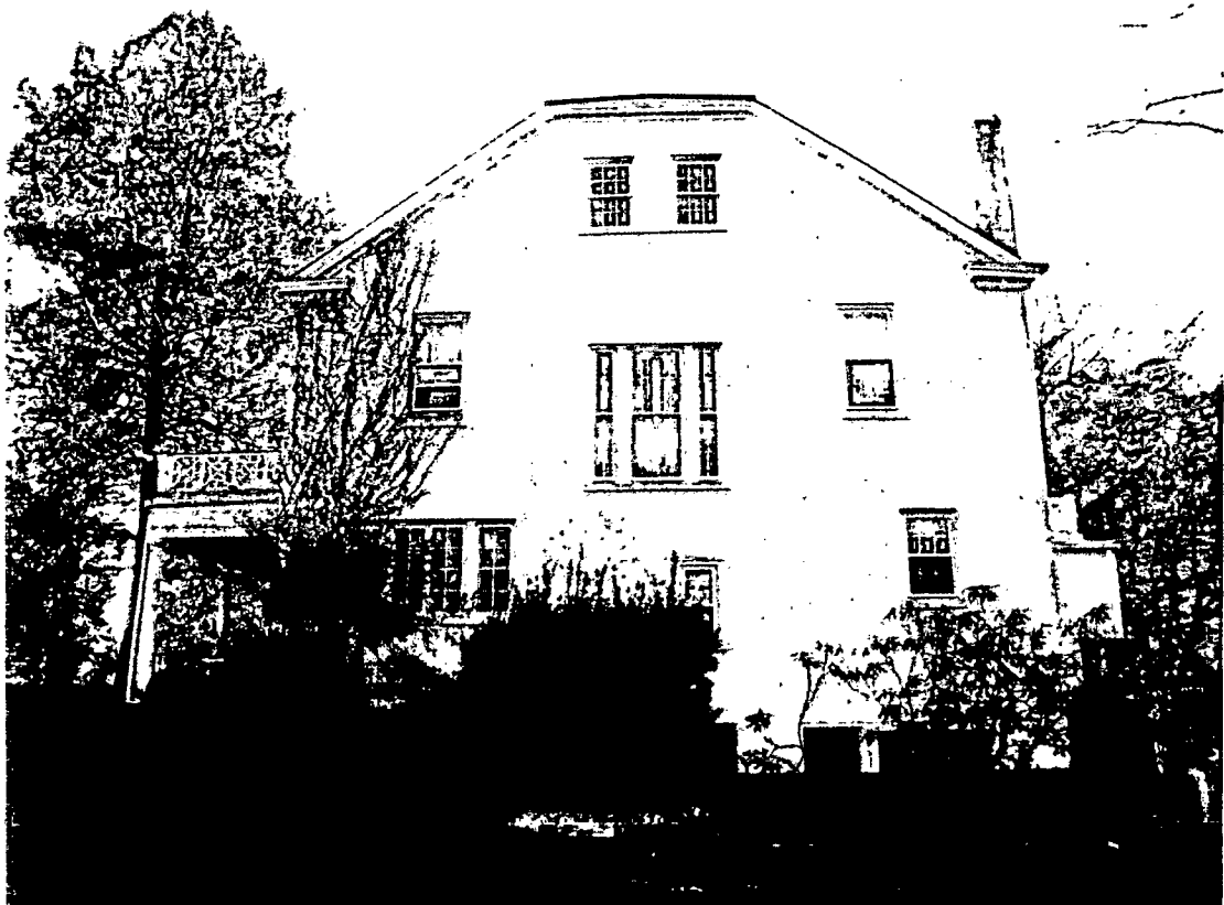
Existing Rear of House
