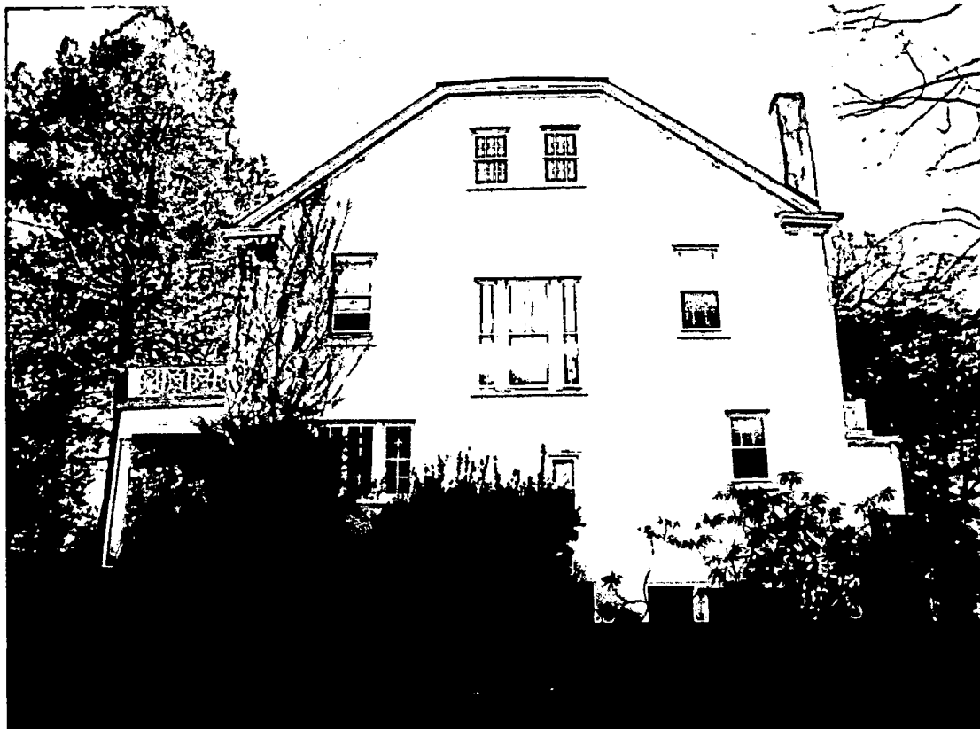
Existing Rear of House
