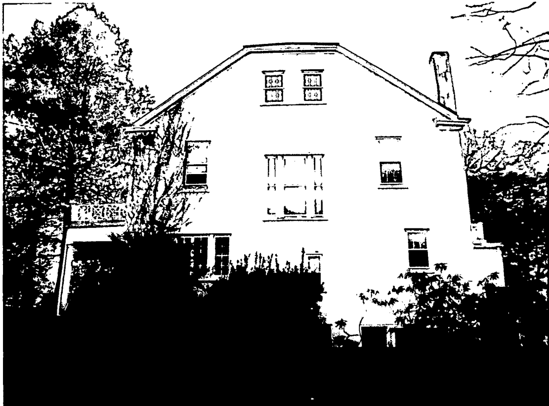
Existing Rear of House
