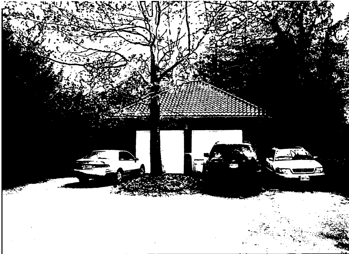
EXISTING GARAGE ON PROPERTY
