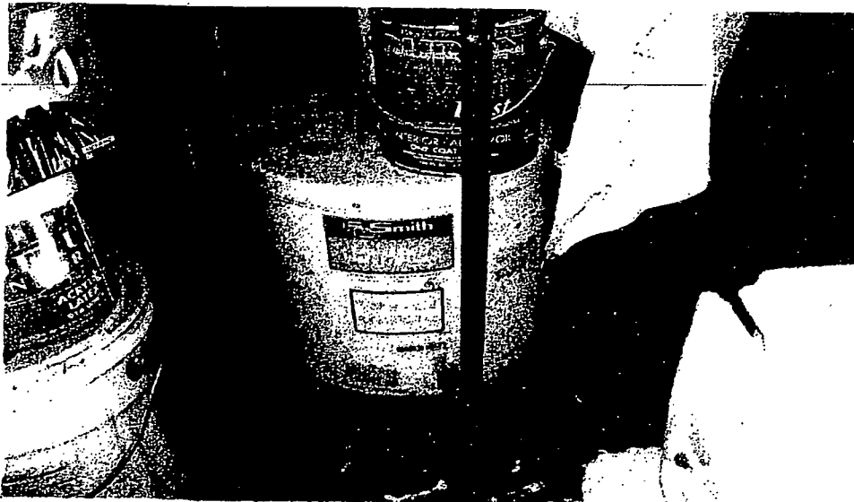
PHOTOGRAPH 2: Non-operational Domestic Water Heater
