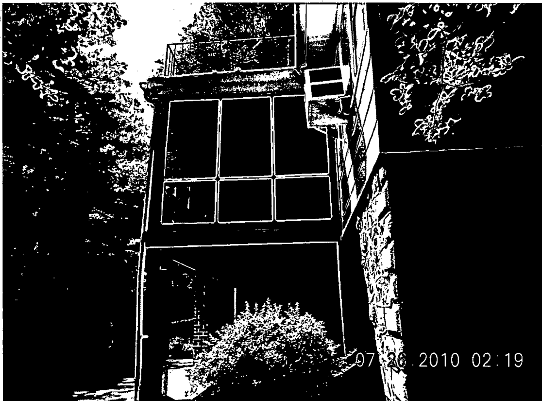
VIEW FROM BACK LEFT CORNER OF HOUSE – REAR PORCH TO BE REMOVED.
