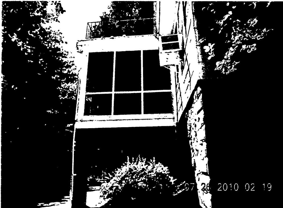
VIEW FROM BACK LEFT CORNER OF HOUSE – REAR PORCH TO BE REMOVED.
