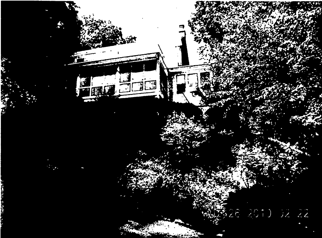
REAR VIEW OF HOUSE FROM MIDDLE OF YARD – ON SLOPE
