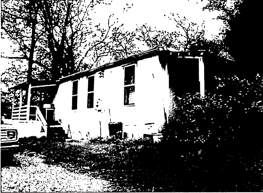
8822 Hawkins Lane, south view
