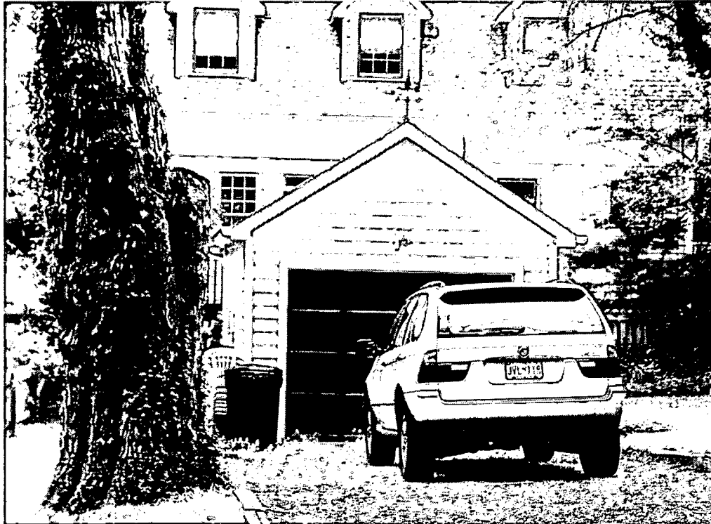
8813 Hawkins Lane, garage
