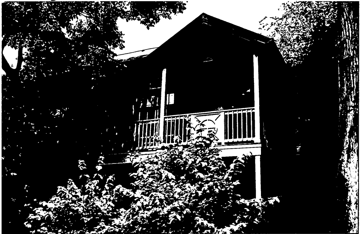
Rear Elevation. New windows will be below deck, at the lower level.
