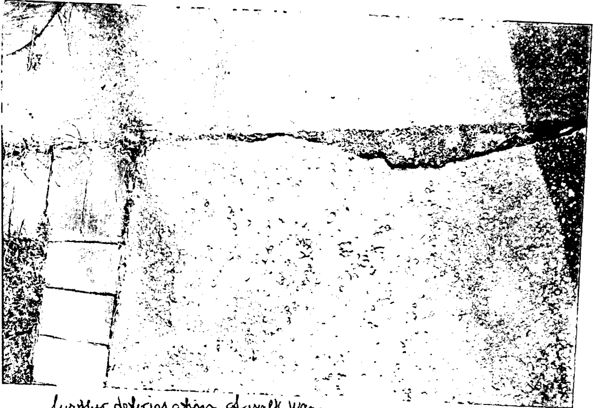
Shows deterioration of walk way
