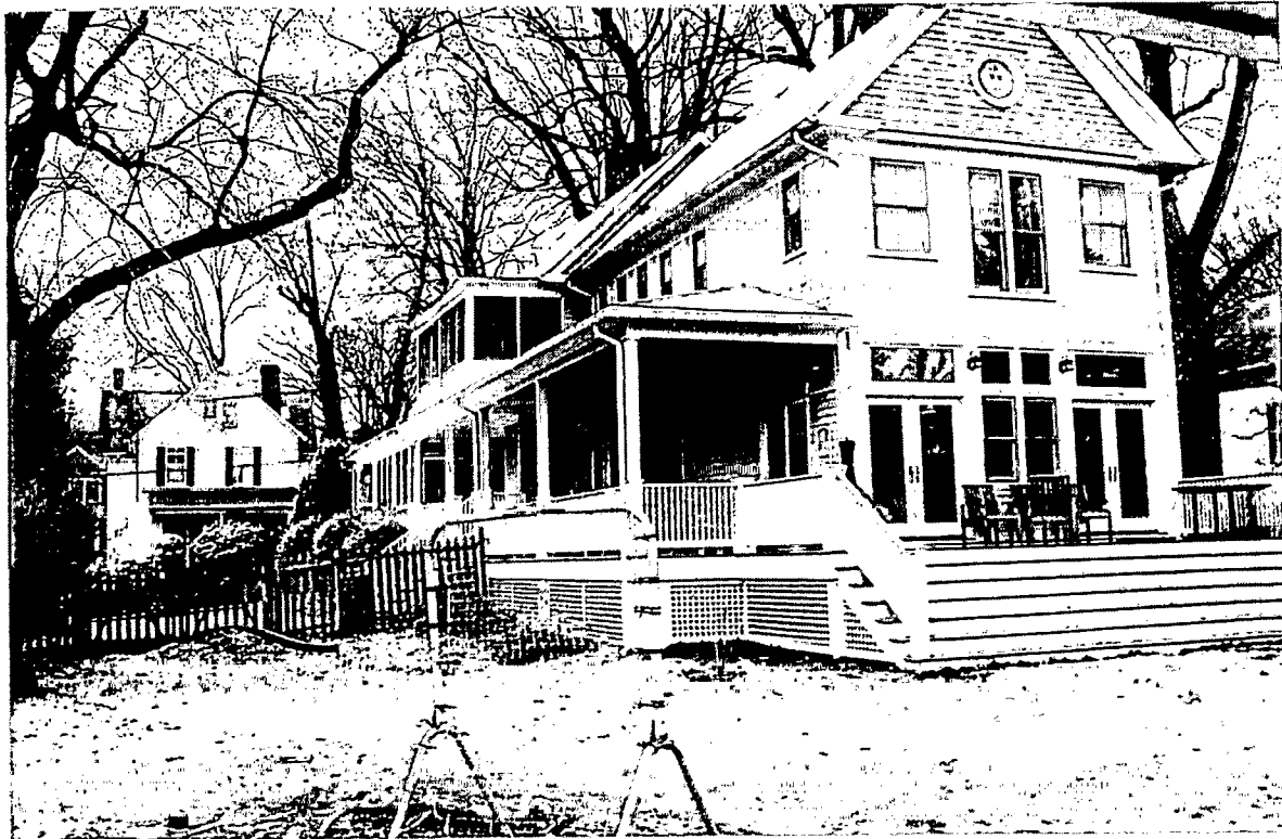
VIEW AT REAR OF HOUSE
