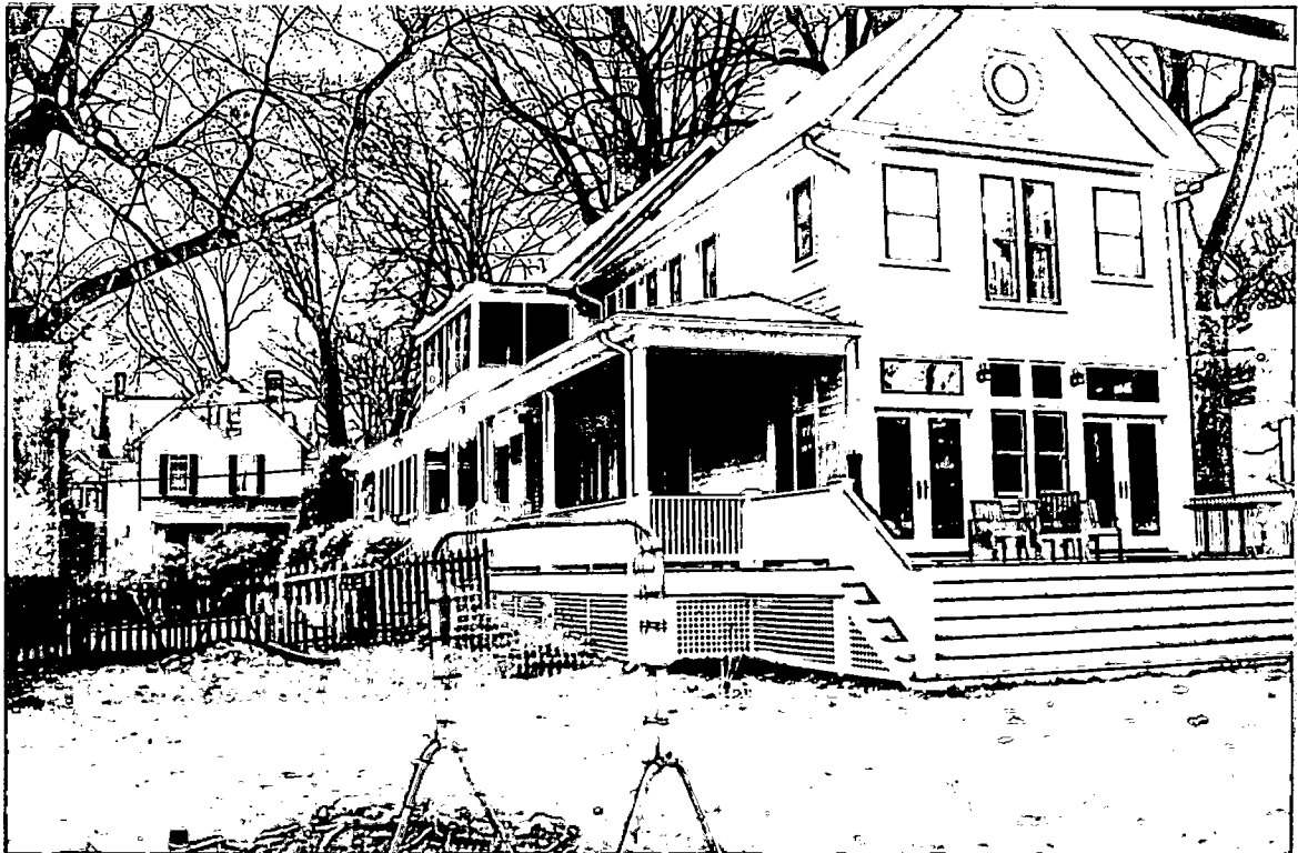
VIEW AT REAR OF HOUSE
