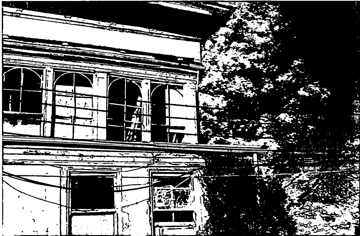
9C Northeast Corner
