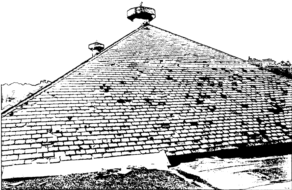
7A Roof – North Side
