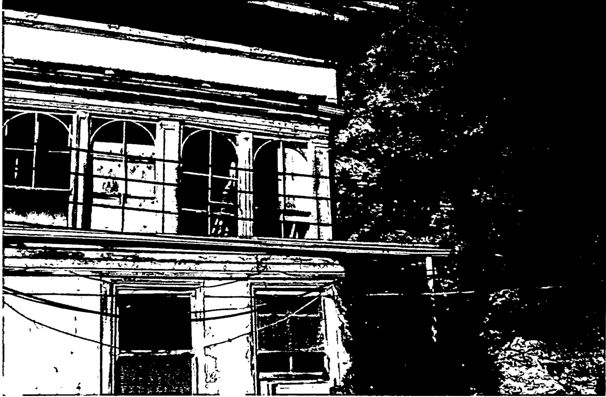
9C Northeast Corner
