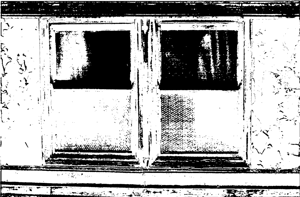
9A Window - East Side
