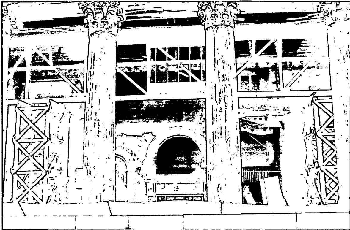
10D West Side – Portico
