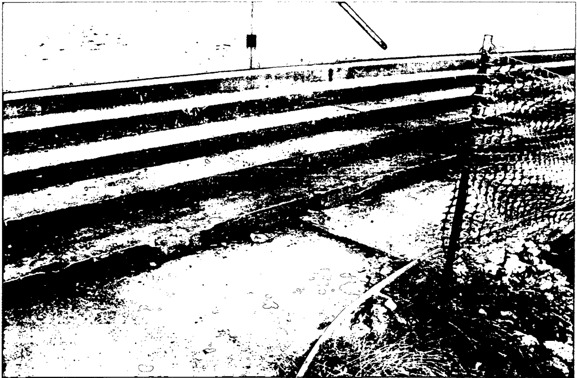
1B Portico Steps – West Side
