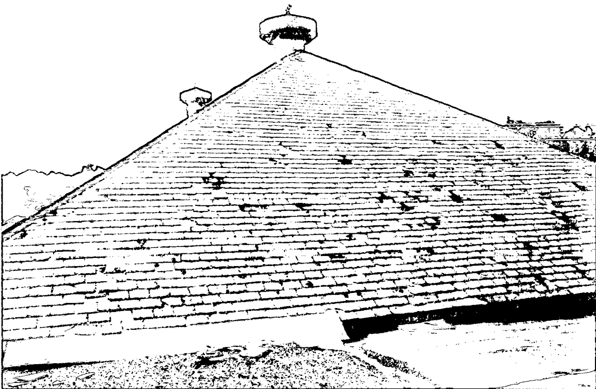
7A Roof – North Side
