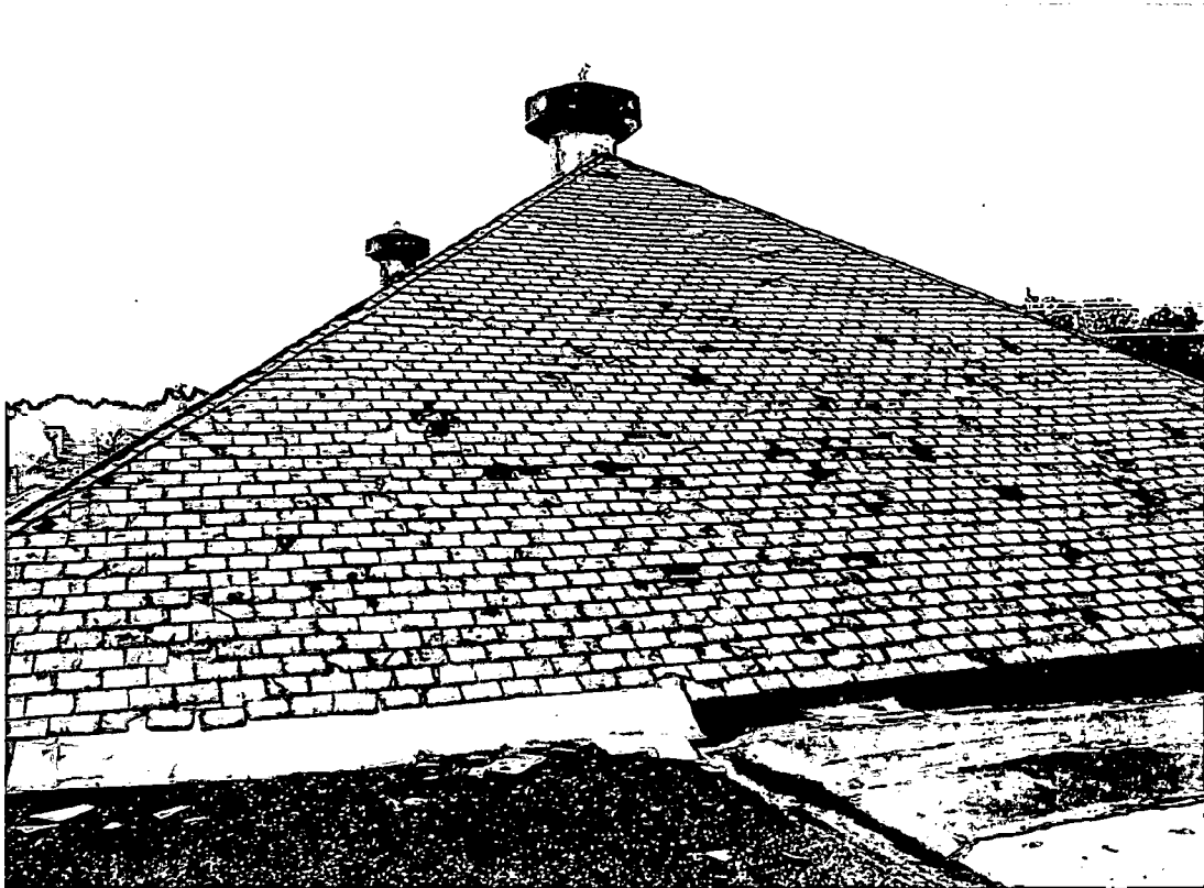
13A- Slate Roof, West Side
