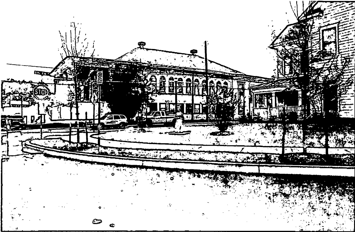
2A- Southwest corner
