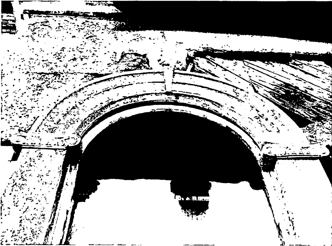
10A- Window Detail, North Side
