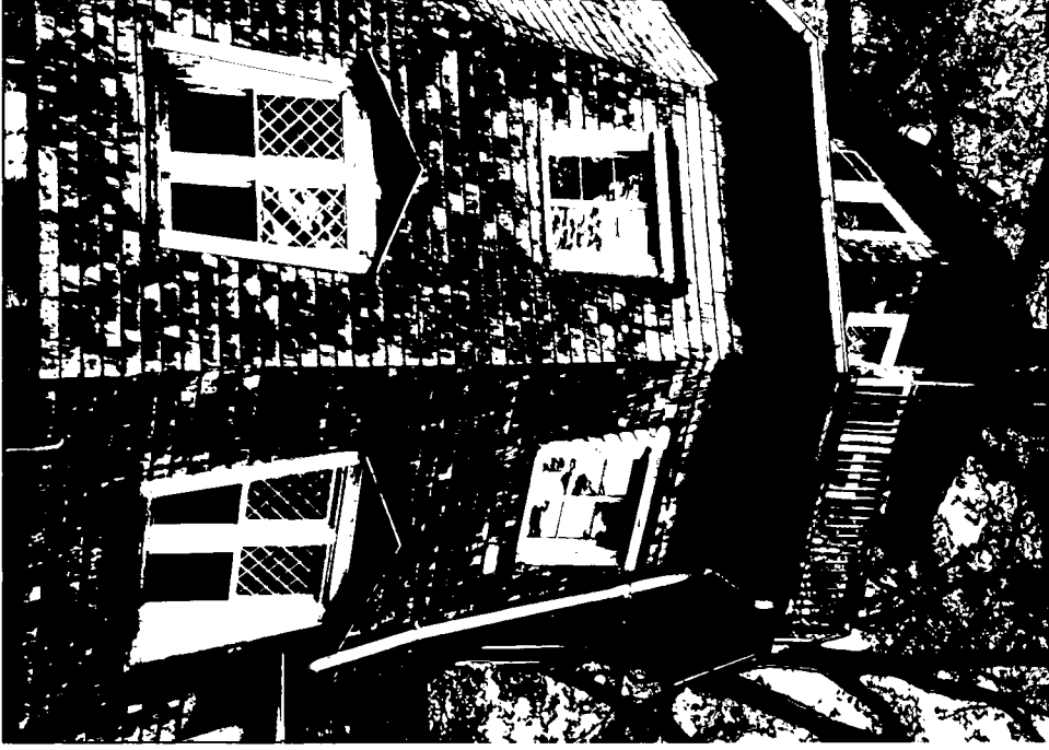
Photo # 4 - storm windows for 1st floor & 2nd floor of tower
