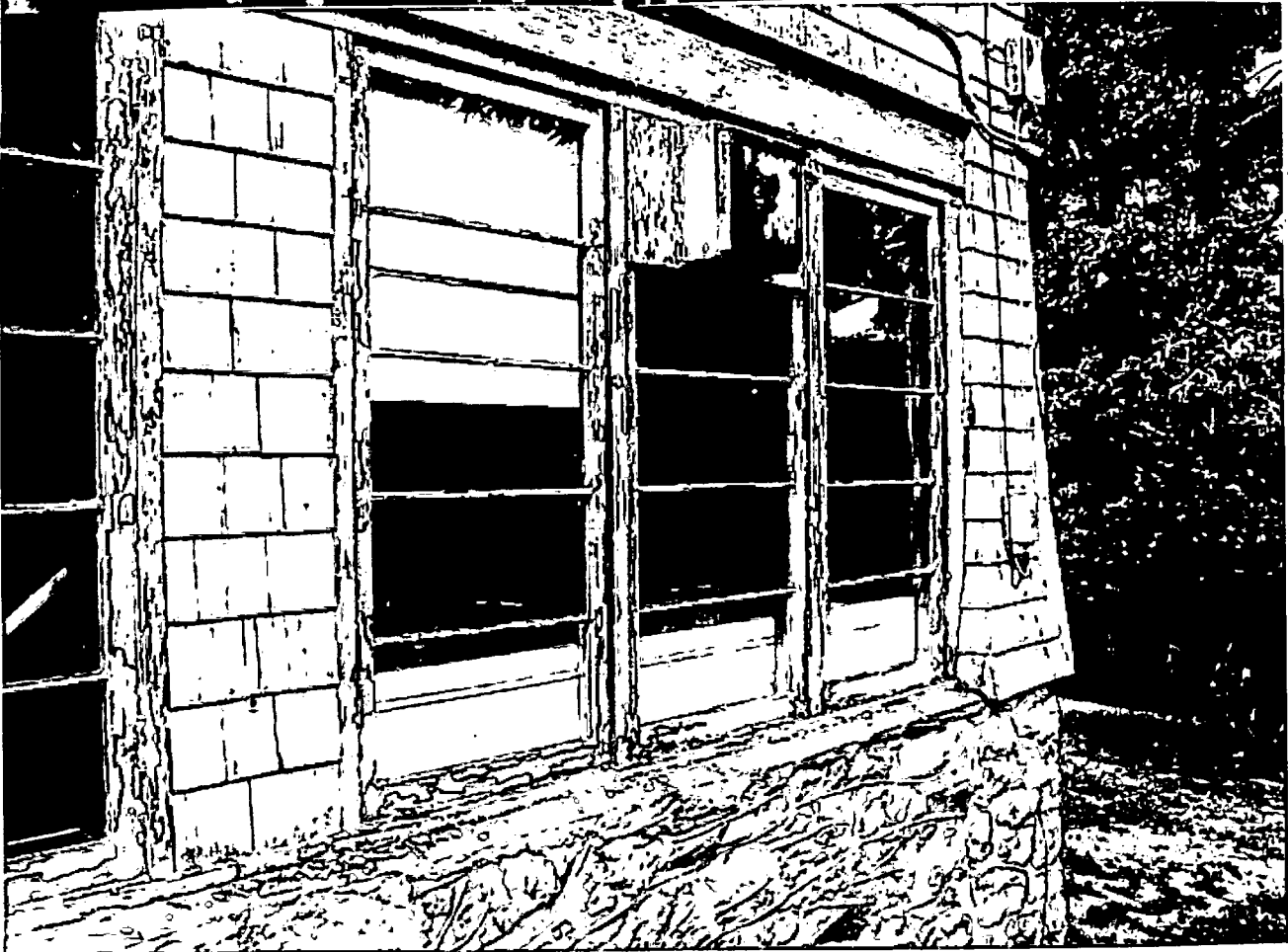
CLOSE-UP VIEW OF REAR OF HOME - INDICATIVE OF WINDOW / PAINT / SHINGLE DETERIORATION
