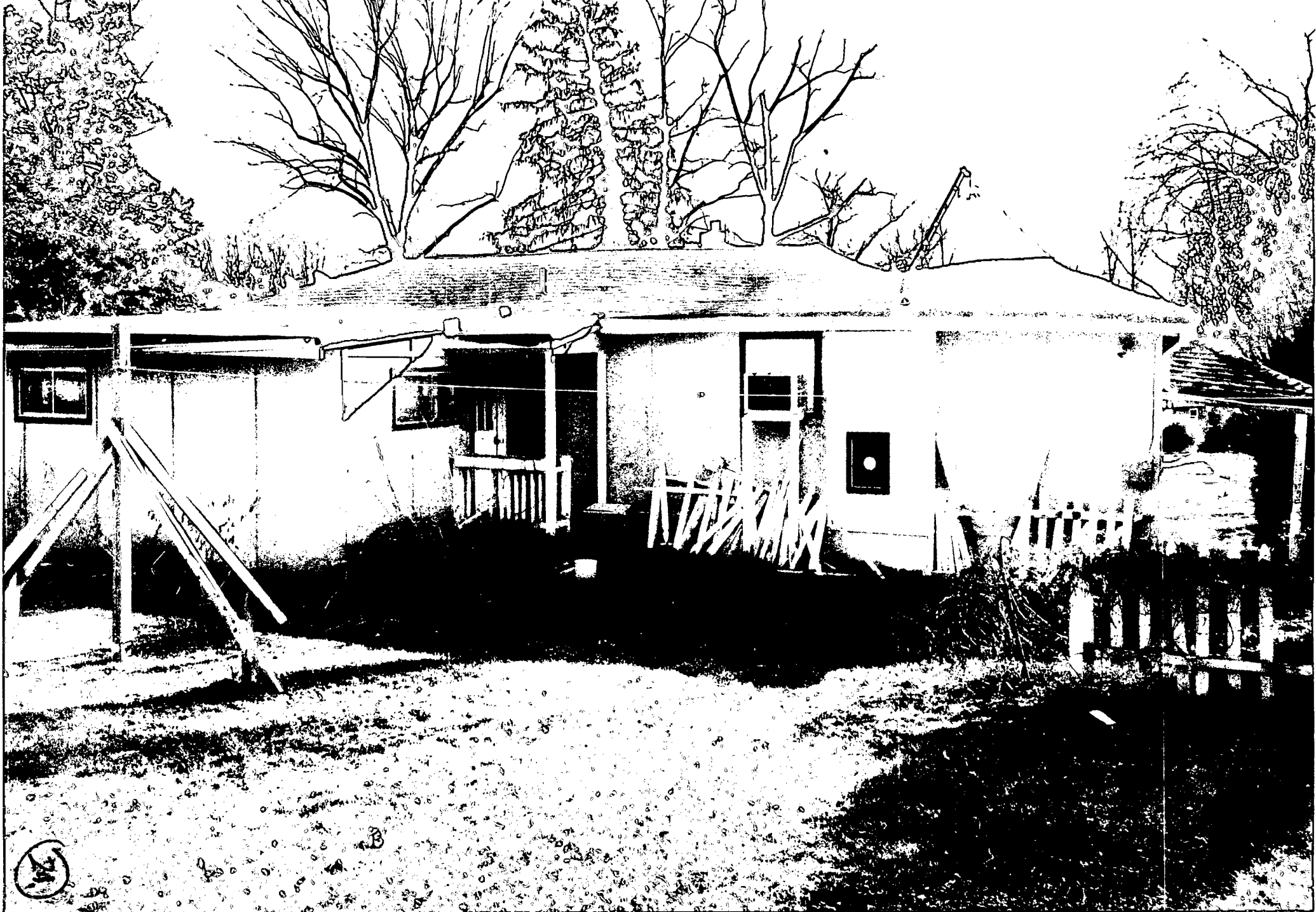
Salisbury Road Property View of Rear (North) Face
