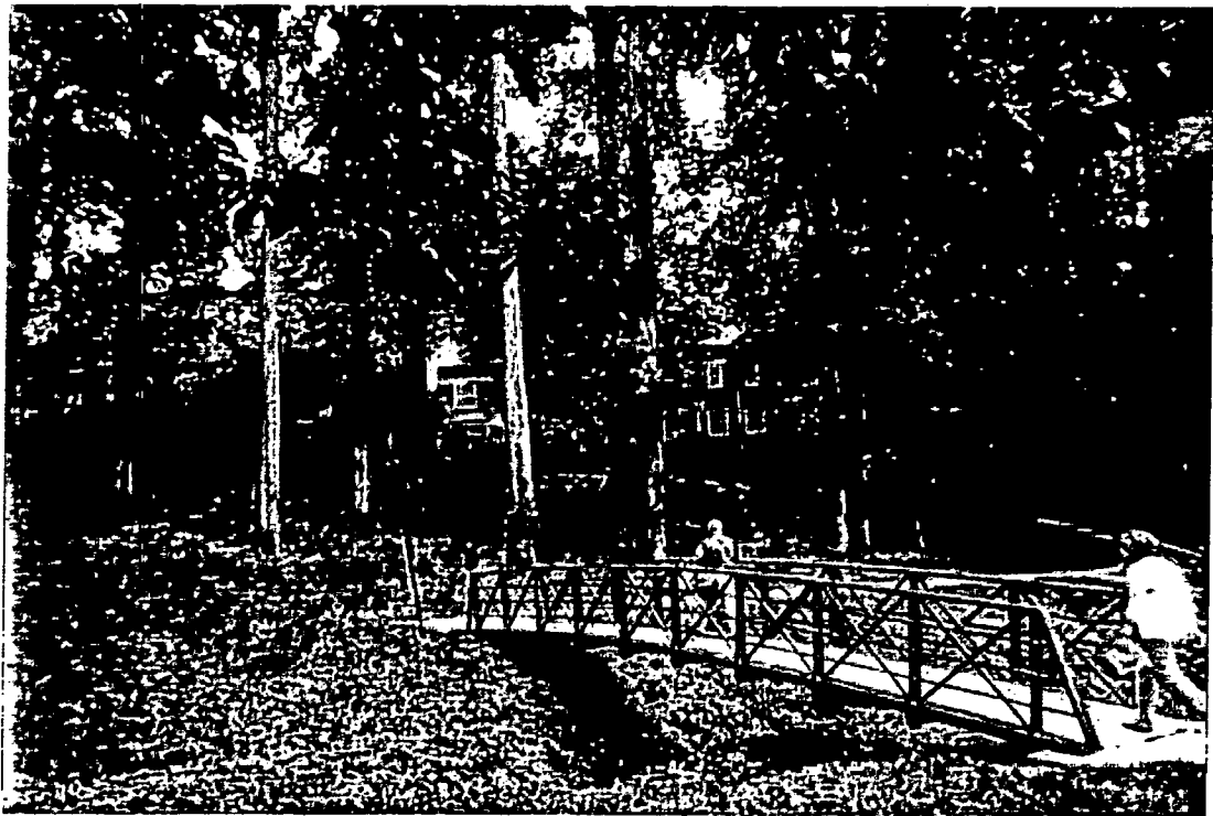
Detail: View 4: Existing pedestrian bridge
