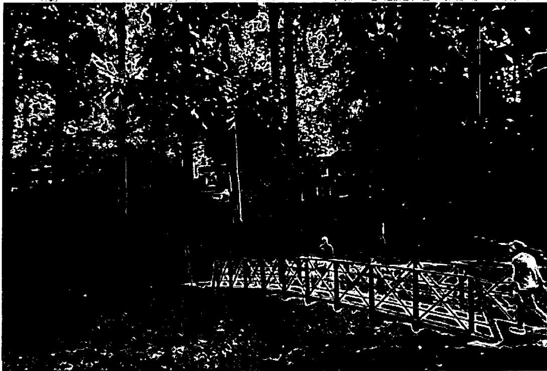
Detail: View 4: Existing pedestrian bridge
