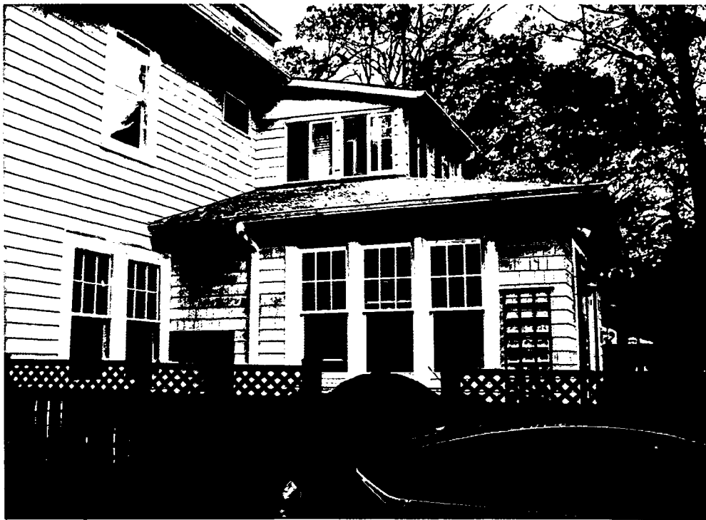
South façade of existing one-story rear addition (built below original sleeping porch ca 2003)
