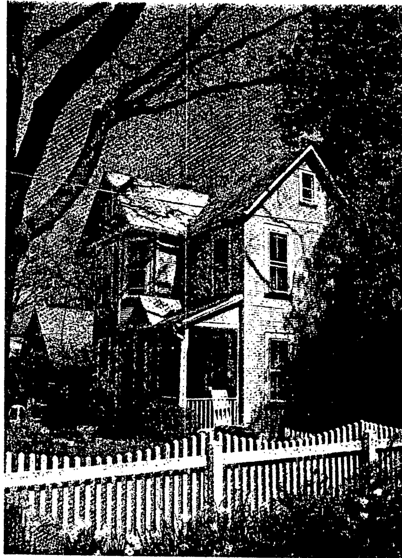
View of West corner of house
