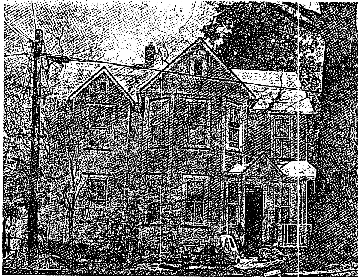
Northwest Elevation (Street Elevation) of House
