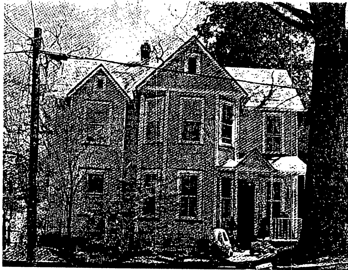
Northwest Elevation (Street Elevation) of House
