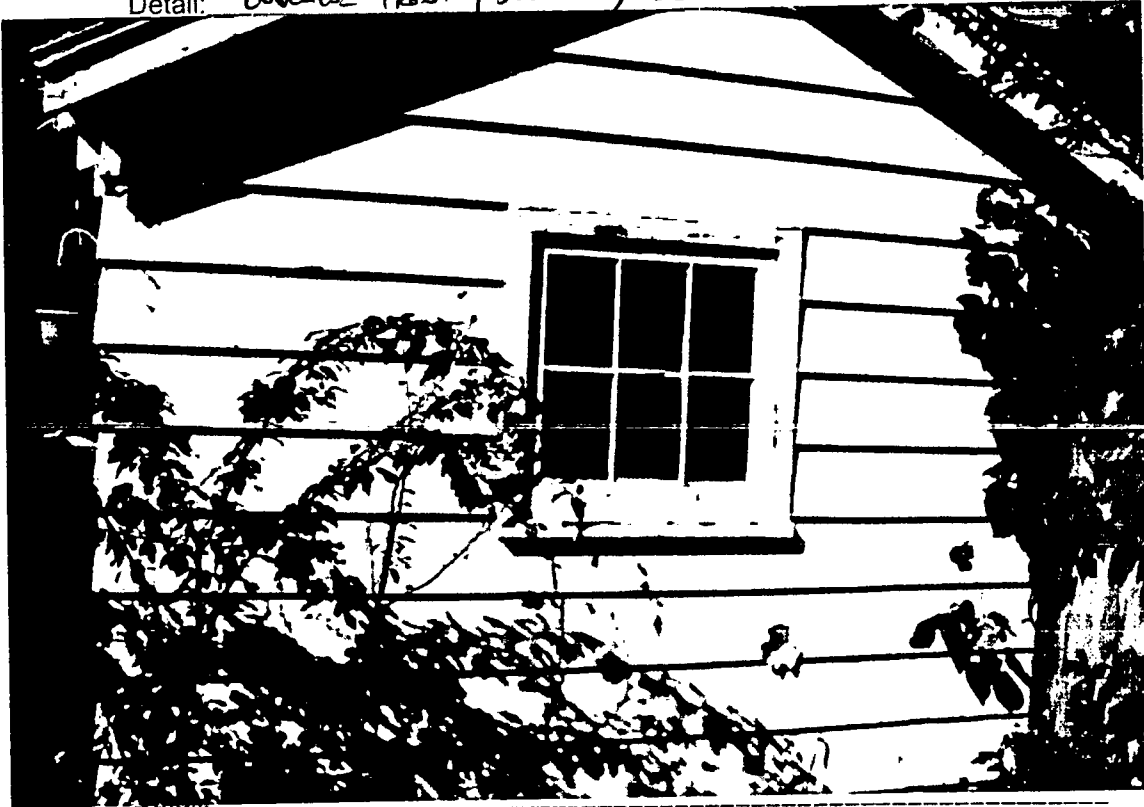
GARAGE REAR (WEST) ELEVATION
