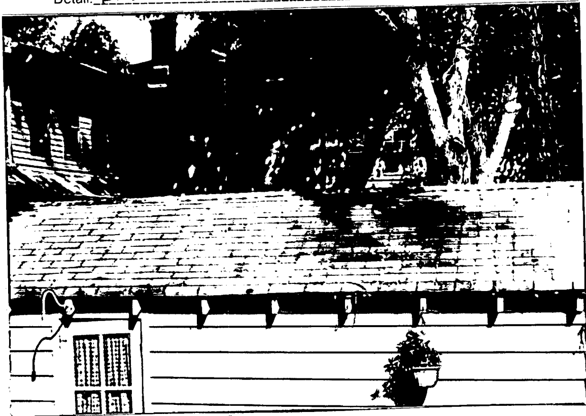
EXISTING ROOF - GARAGE
